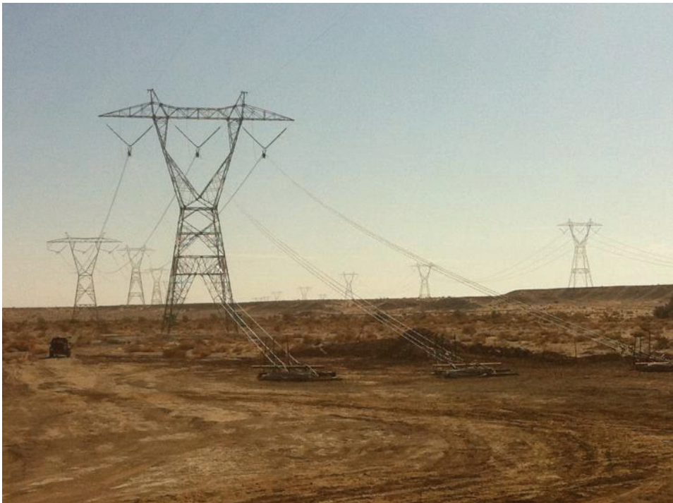
Figure 1: Wire and snubs at EP322/EP323 pull site. Temporary mats have been removed. (Link 1)
