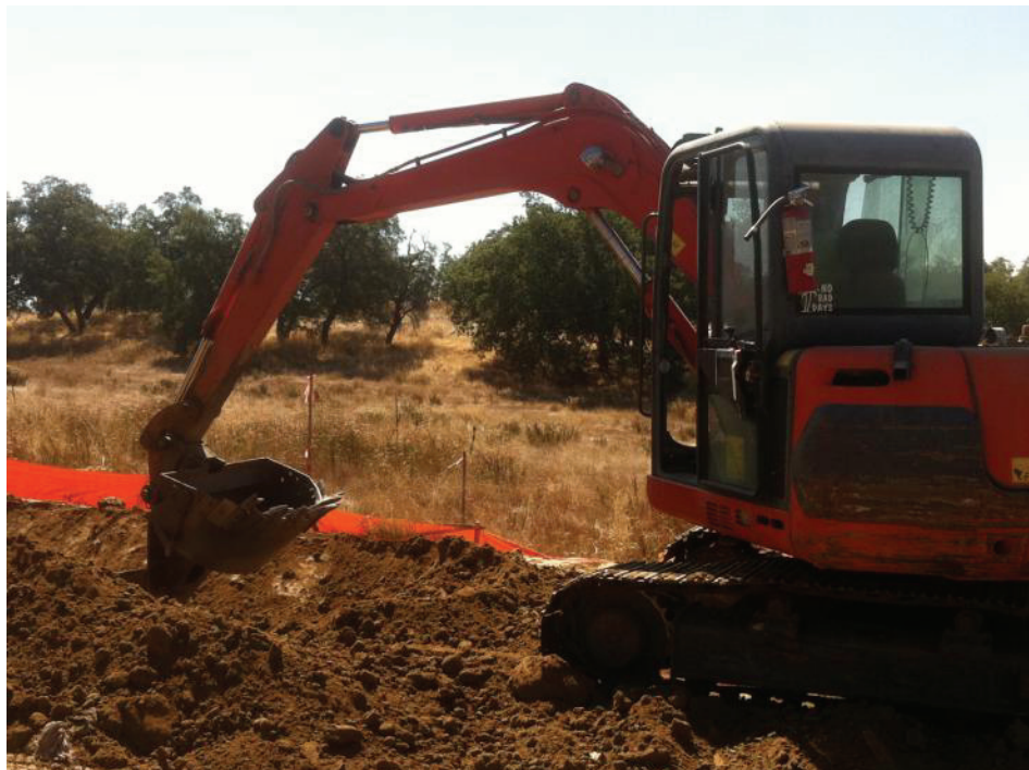
Figure 10: Trenching between vaults for underground utilities along BBTT. (Link 3)
