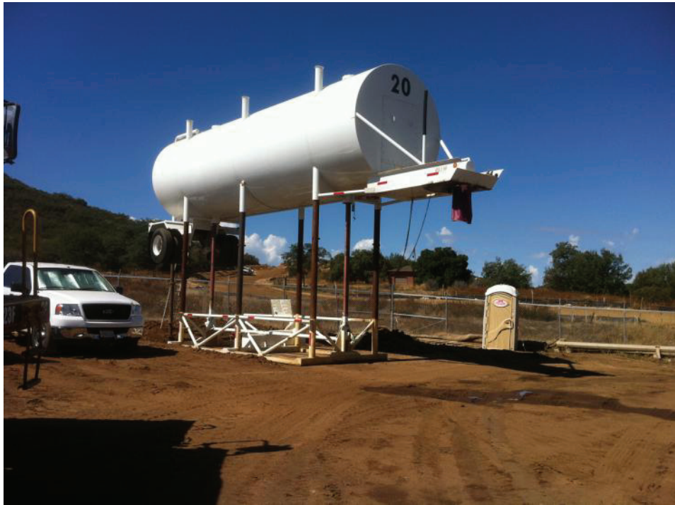
Figure 11: Water tank installed at Wilson Yard. (Link 3)
