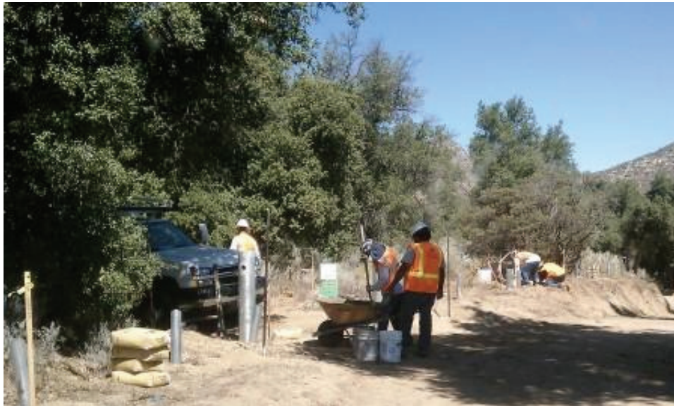
Figure 3: Installation of gate posts along La Posta Road. (Link 2)
