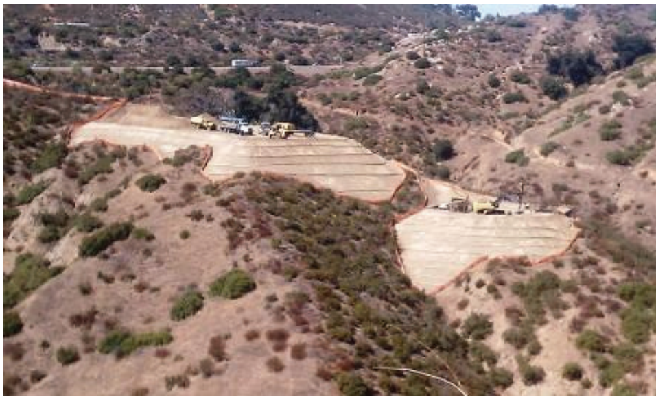
Figure 4: Conventional drilling at CP87-1 (right) with pull site above. (Link 5)
