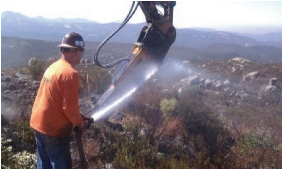
Figure 5: Breaking boulders and wetting vegetation at CP100-1. (Link 5)
