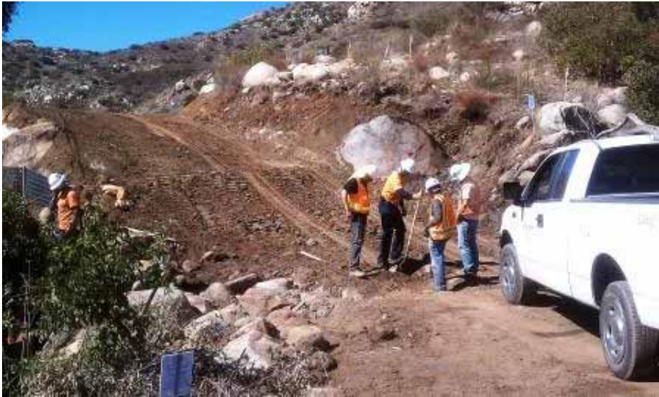
Figure 1: Culvert installation along access road to Barrett Construction Yard. (Link 2)
