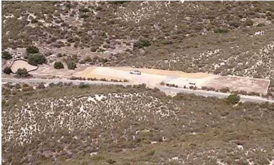
Figure 2: Helicopter view of pullsite in USFS land, south of EP125. (Link 2)
