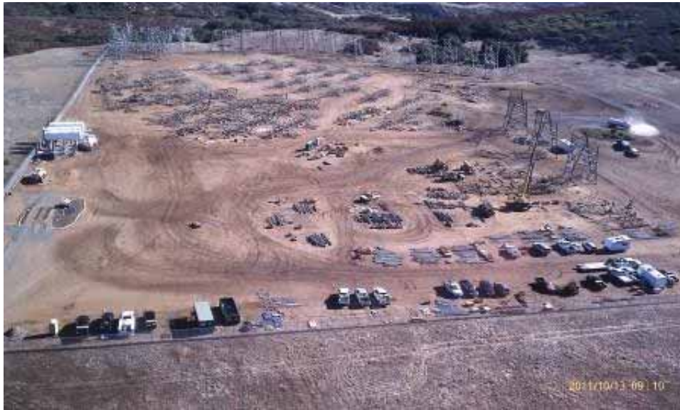
Figure 5: View from helicopter of SWAT Construction Yard. (Link 2)
