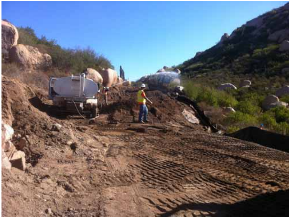
Figure 3: Grading the access road to CP100-1. (Link 5)
