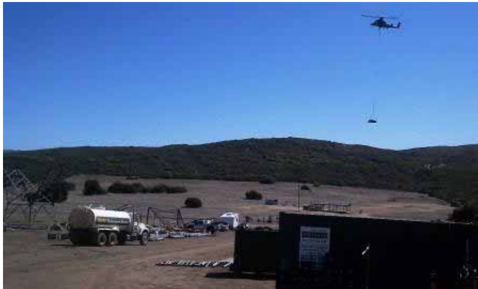
Figure 4: Helicopter operations at Bartlett Hauser Construction Yard. (Link 2)
