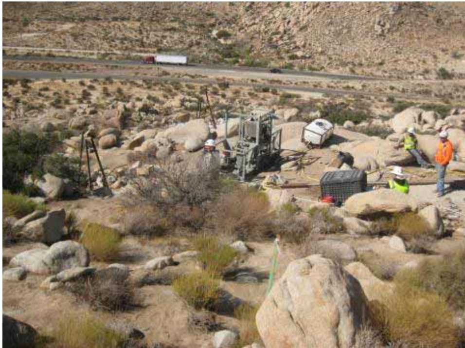
Figure 2: Micropile activities at EP261. (Link 1)
