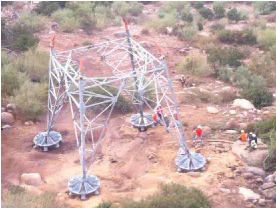
Figure 14: Assembled legs at CP65-1. (Link 5)
