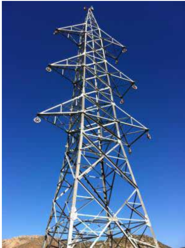
Figure 13: Completed tower at CP75-1. (Link 5)
