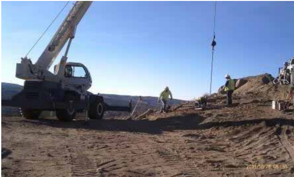
Figure 9: Setting cages at EP131. (Link 2)
