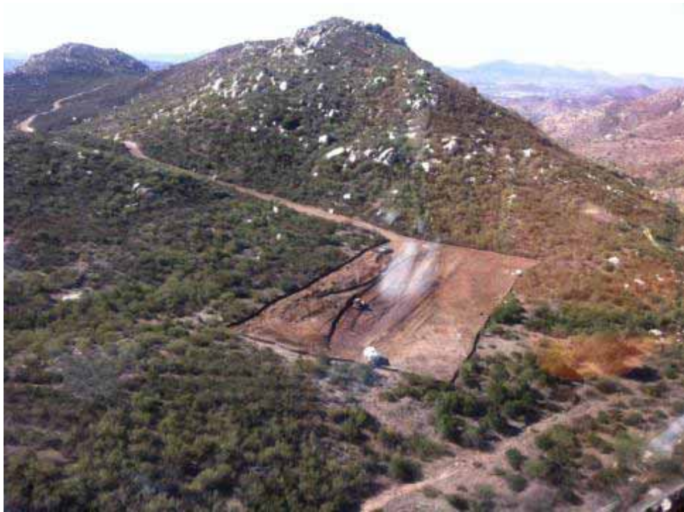
Figure 11: Grading at CP55/CP56-1 pull site. (Link 5)
