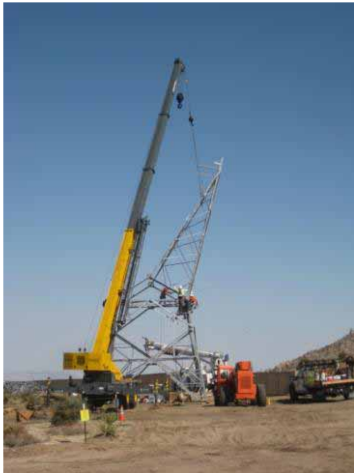
Figure 16: Crews assembling tower sections at Fromm Yard. (Link 1)
