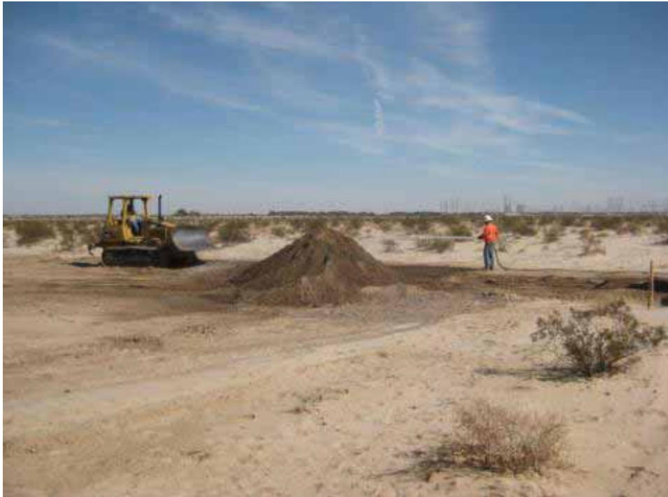
Figure 18: Crews restoring IV Substation Yard. (Link 1)
