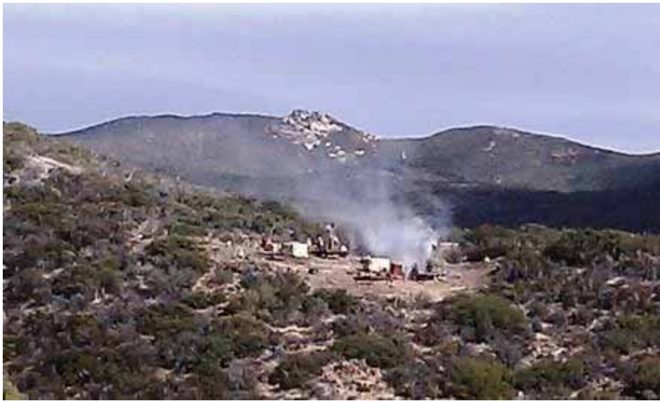
Figure 8: Micropile drilling at EP139. (Link 2)
