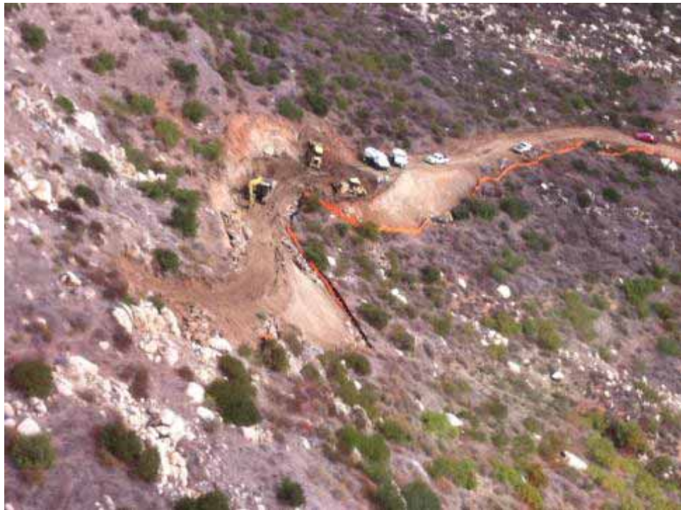
Figure 12: Access road grading to CP49-1 pull site. (Link 5)
