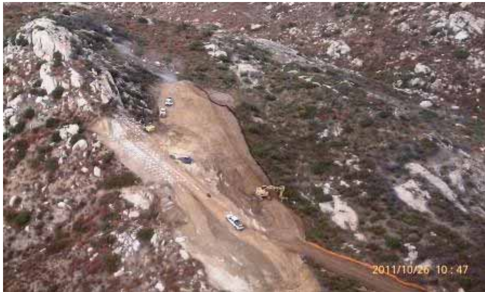
Figure 4: EP47 and pullsite viewed from helicopter. (Link 2)
