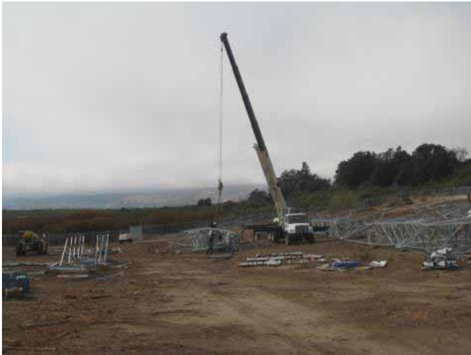
Figure 17: Crews assembling tower components at S2 Yard.
