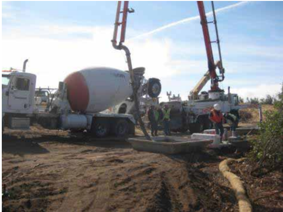
Figure 3: Concrete operations at EP180. (Link 1)
