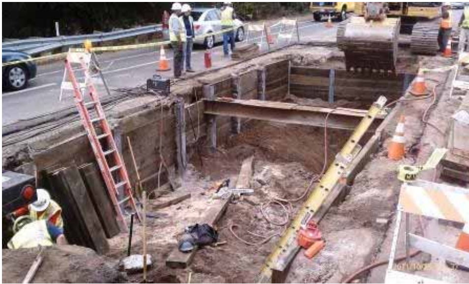
Figure 10: Excavating bore pit at Alpine Creek. (Link 4)
