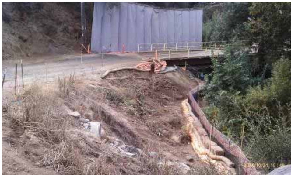
Figure 15: Bauer Bridge and stormwater BMPs. (Link 4)
