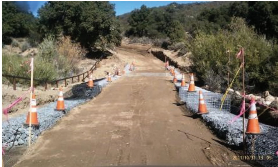
Figure 7: Culvert installation at La Posta Road. (Link 2)
