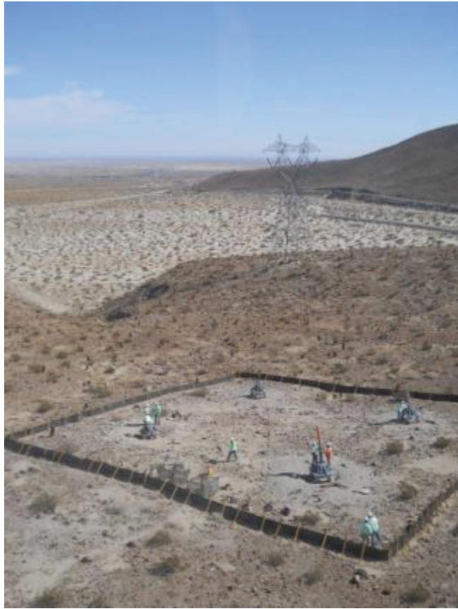
Figure 2: Tower assembly activities at EP280. (Link 1)
