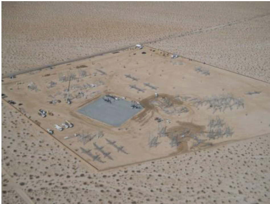
Figure 13: Aerial view of S-2 Yard. (Link 1)
