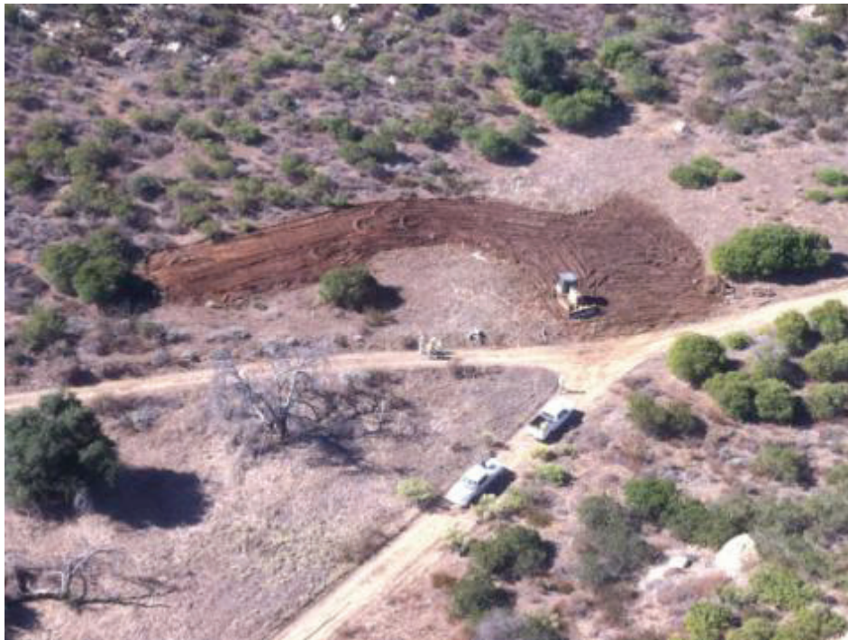
Figure 9: Grading at CP31-2 pull site. (Link 5)
