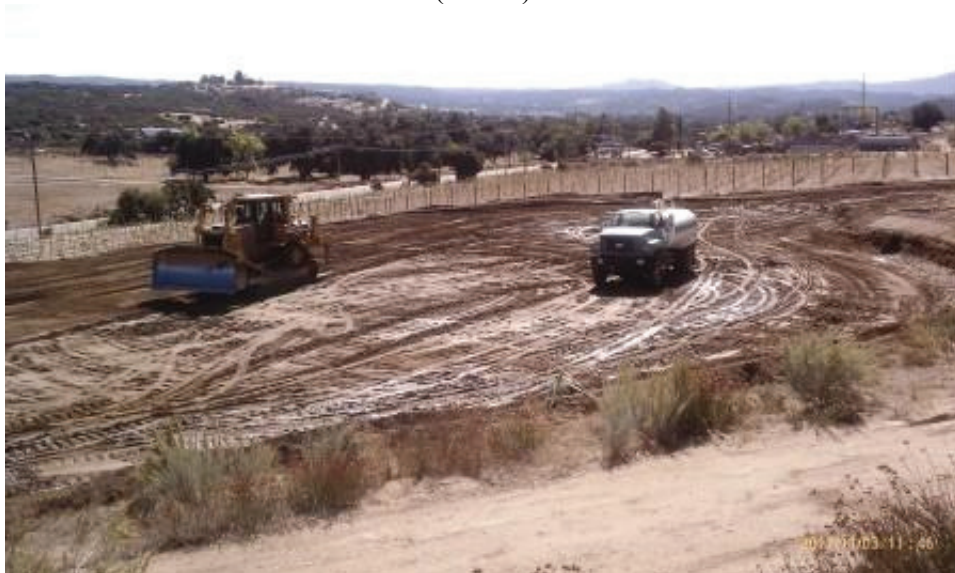
Figure 3: Grading of EP89 pull site. (Link 2)
