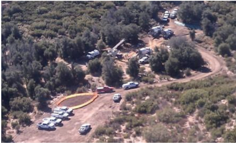
Figure 8: EP141 pull site in foreground; concrete being poured at EP141. (Link 2)
