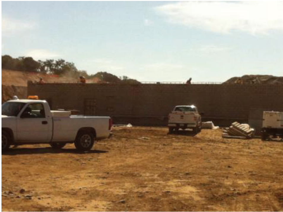
Figure 12: Setting concrete blocks for control shelter. (Link 3)
