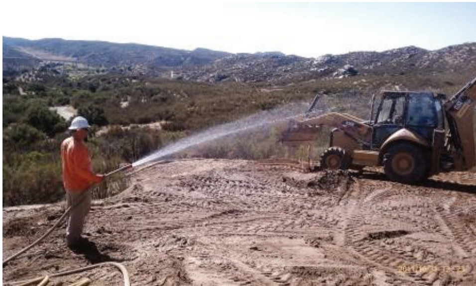
Figure 5: Grading and watering at EP126. (Link 2)
