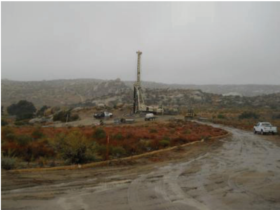
Figure 1: Conventional foundation crews working during rain event at EP198. (Link 1)
