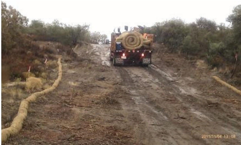
Figure 4: BMP truck making ruts attempting to go uphill on access road to EP105. (Link 2)
