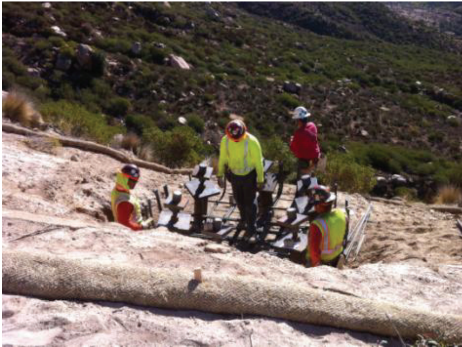
Figure 10: Micropile cap work at CP67-3. (Link 5)
