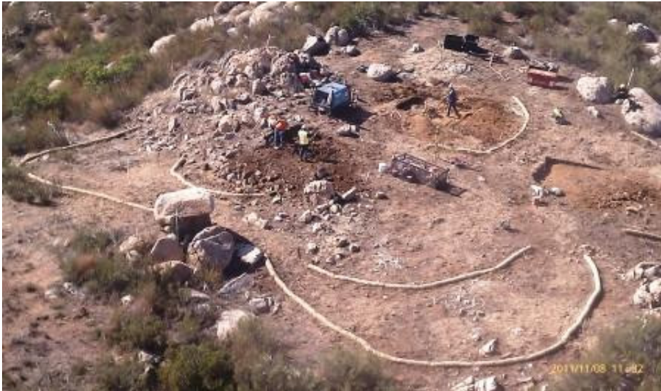
Figure 2: Micropile preparation work at EP6-1. (Link 2)
