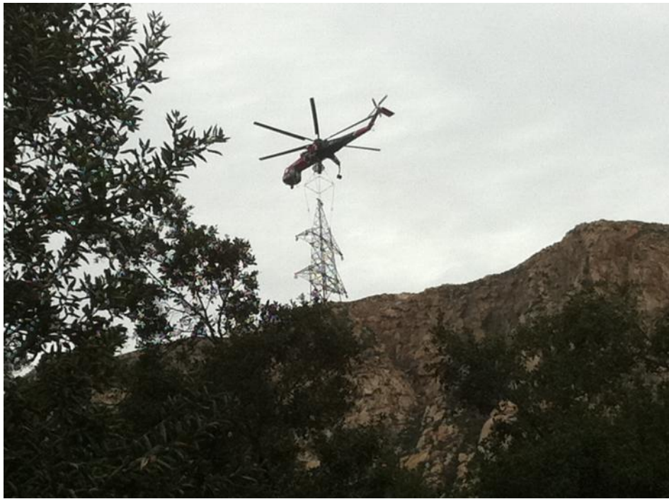
Figure 5: Aircrane setting tower at CP67-3. (Link 5)
