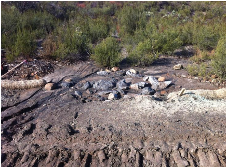
Figure 8: Breached BMPs along access road to CP100-1. (Link 5)
