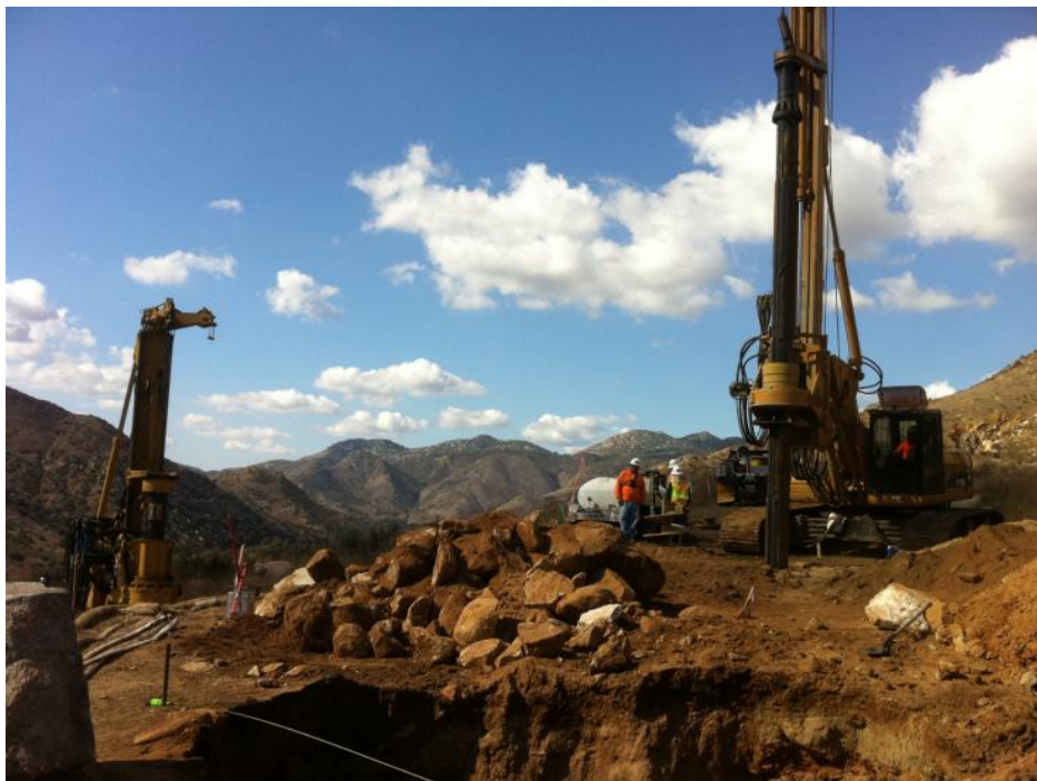
Figure 6: Drilling operations at CP69-2. (Link 5)
