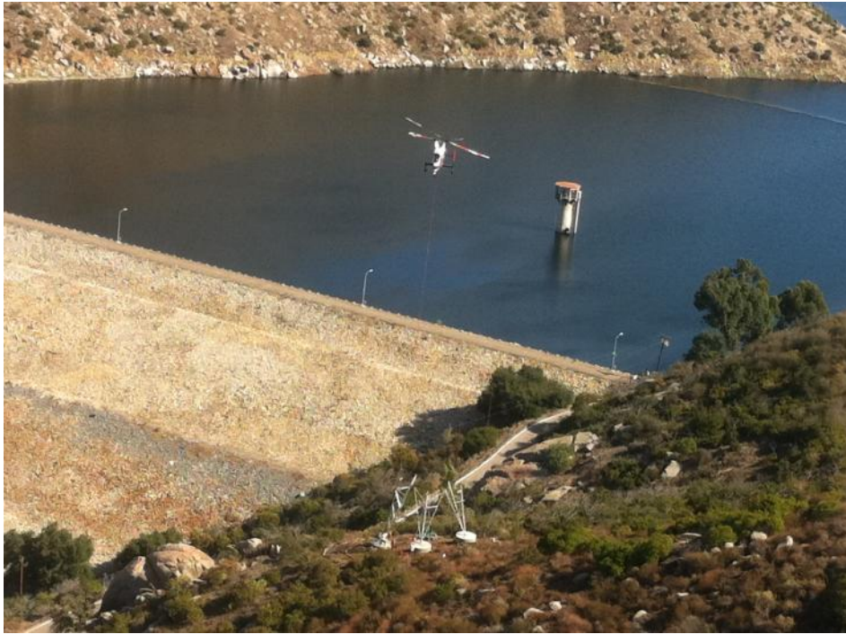
Figure 3: KMAX assembling legs at CP71. (Link 5)
