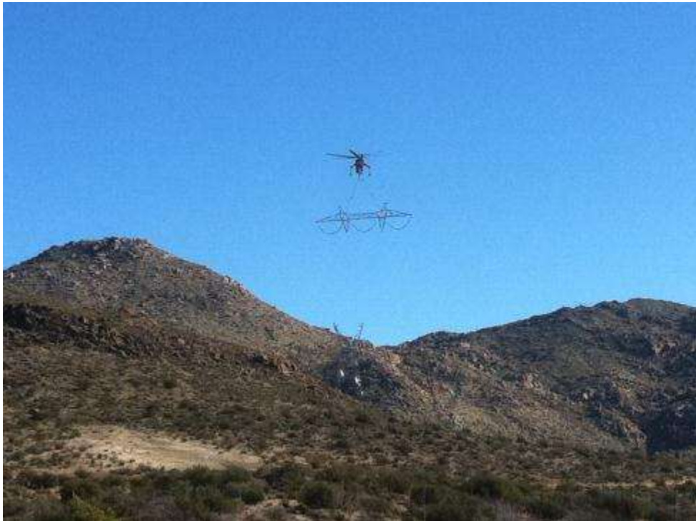
Figure 4: Aircrane setting bridge at EP253-3. (Link 1)
