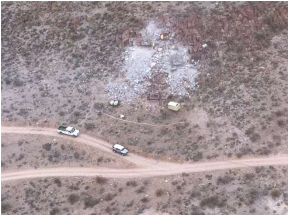
Figure 1: Micropile drilling at EP254-3. (Link 1)
