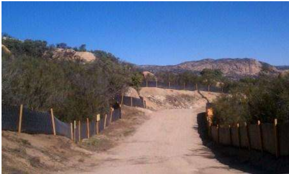
Figure 5: Arroyo Toad fencing installed along access road near EP65. (Link 3)
