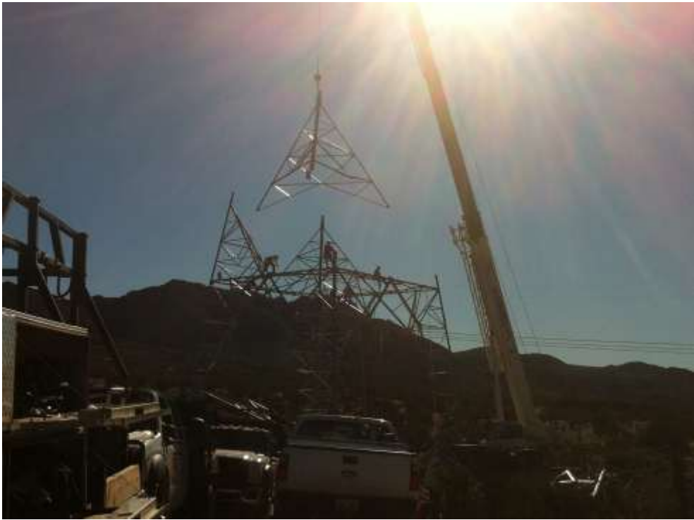
Figure 2: Conventional tower assembly at EP252-1. (Link 1)
