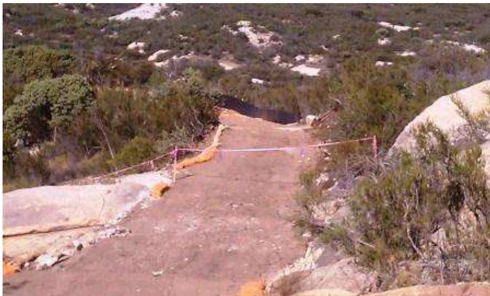
Figure 6: Access road to EP58-2 closed due to USFS-related work shutdown. (Link 2)
