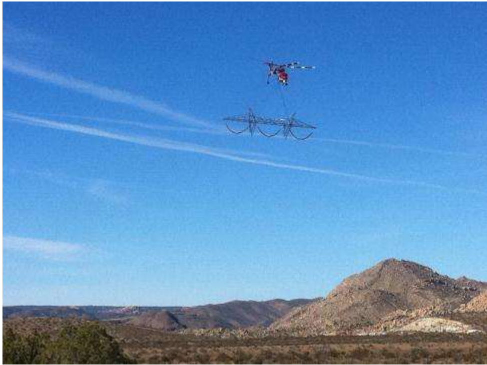
Figure 3: Aircrane flying bridge to EP253-3. (Link 1)
