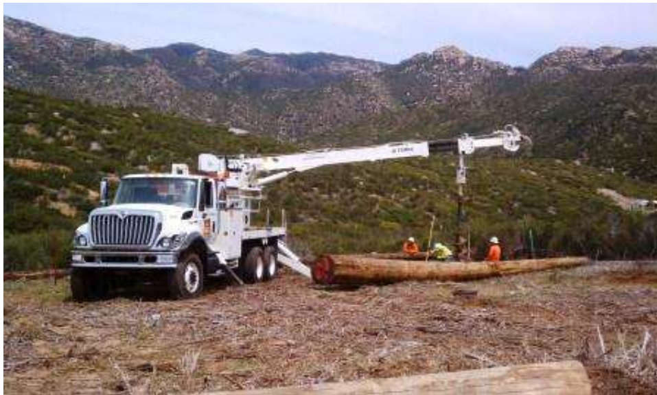
Figure 7: Installation of GS-USFS-2. (Link 2)
