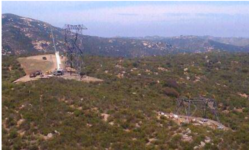
Figure 2: View of Tower EP8-2 (front right) and EP9-1 (left). (Link 2)
