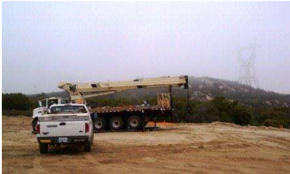
Figure 4: EP83 south pull site with Tower EP83 in background. (Link 2)
