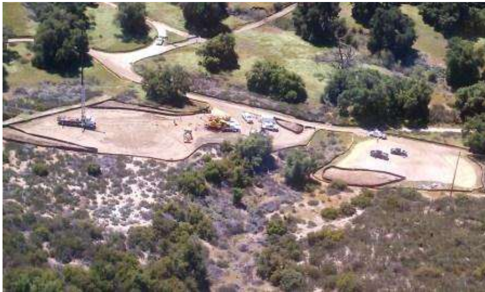
Figure 5: Pull site at Tower EP78. (Link 2)
