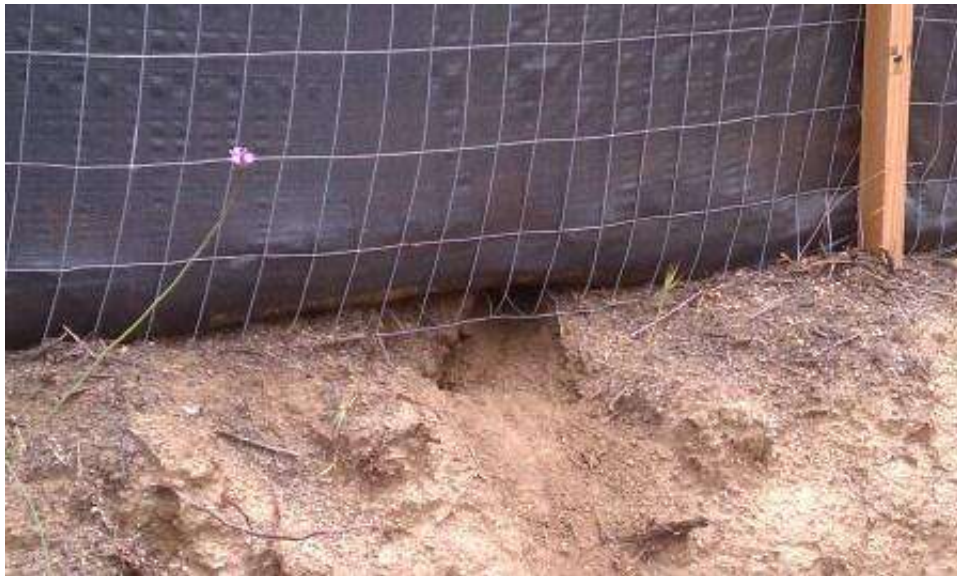
Figure 9: One of several holes in Arroyo toad fence along EP76 access road prior to rain event. (Link 2)
