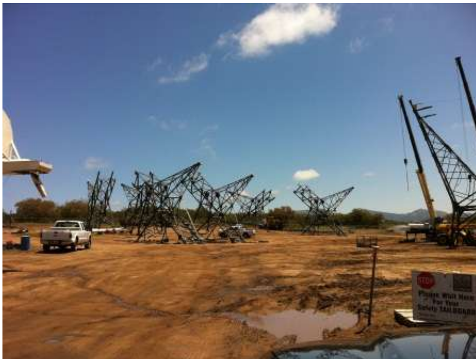
Figure 10: Tower assembly at Wilson Yard. (Link 3)
