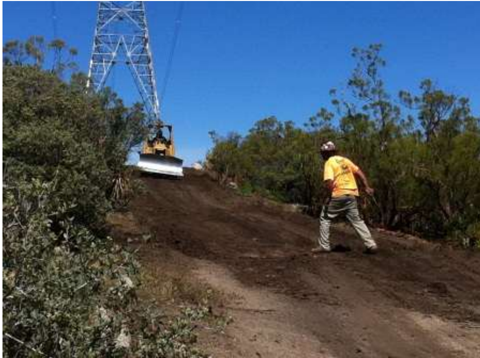
Figure 1: Final road grading at EP186-1-N. (Link 1)
