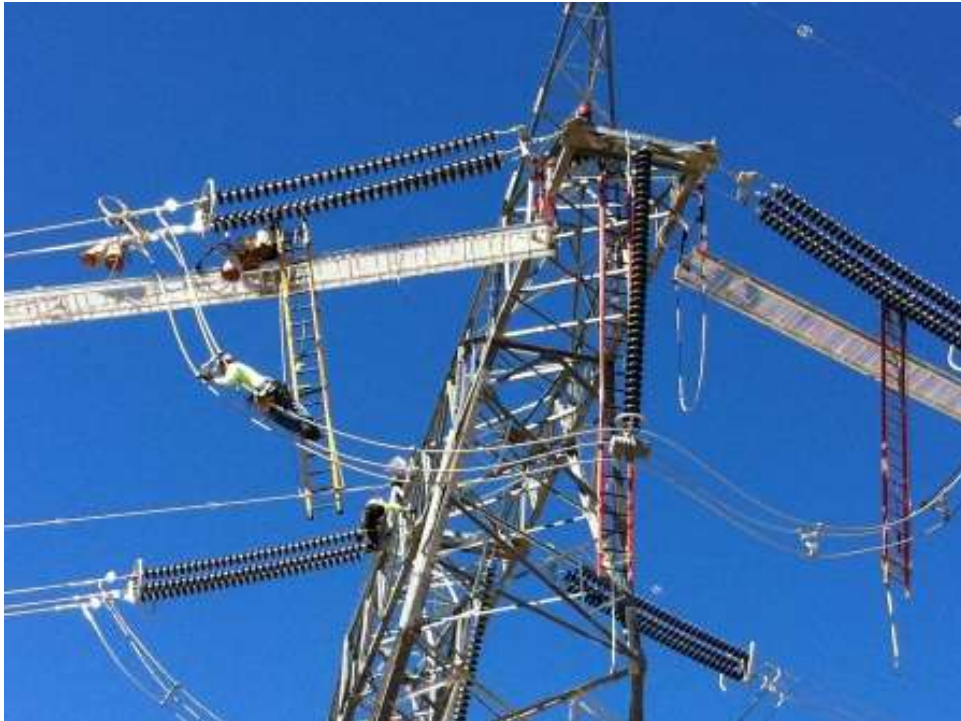
Figure 2: Installing jumpers at Tower EP200-3. (Link 1)
