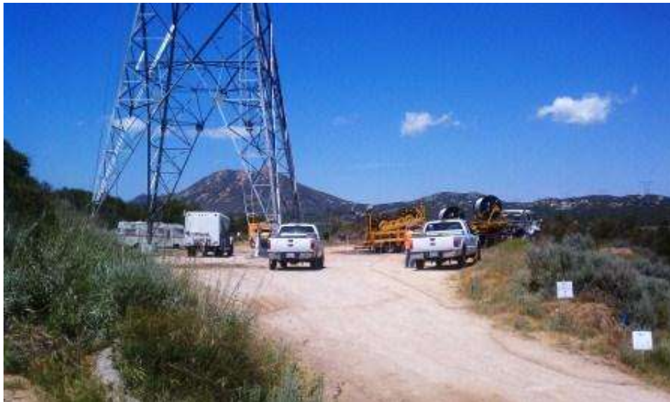
Figure 4: Setting up equipment to pull wire at EP89 pull site. (Link 2)
