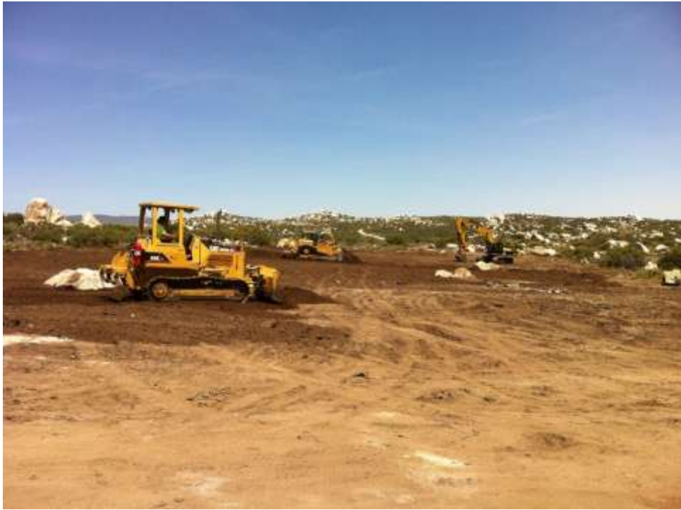
Figure 2: Final grading at EP187-2 pull site. (Link 1)
