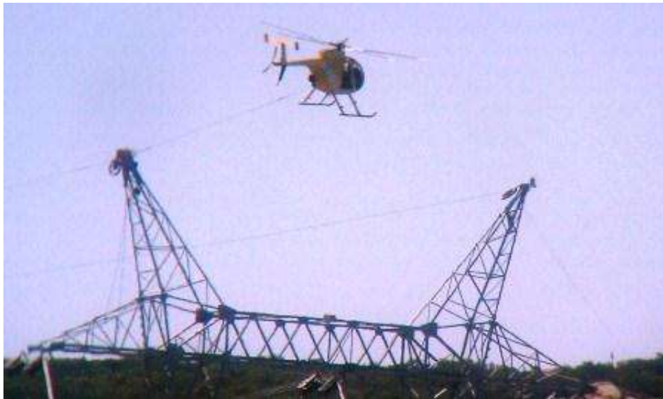
Figure 5: Helo pulling sock line at EP83. (Link 2)
