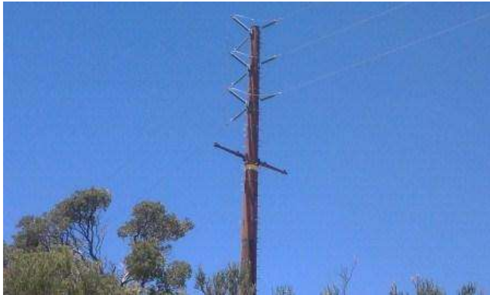
Figure 6: 69 kV pole near EP62A-1 completed. (Link 2)
