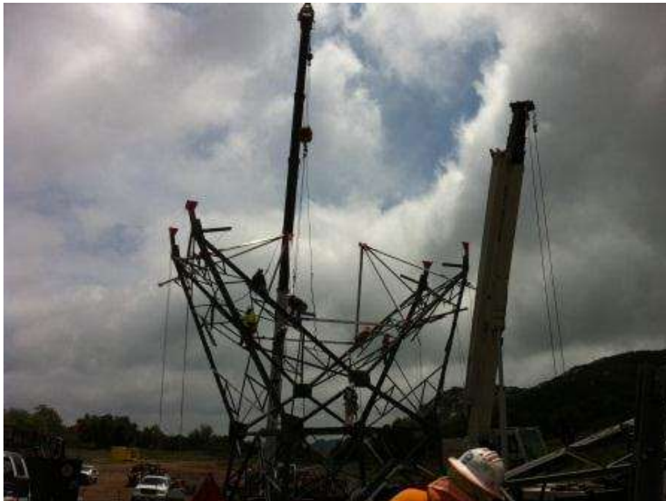
Figure 8: Tower assembly at Wilson Yard. (Link 3)
