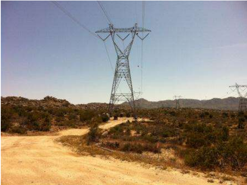
Figure 1: Fiber splicing at Tower EP244. (Link 1)
