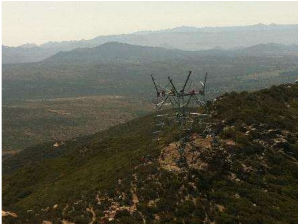
Figure 3: Tower erection at EP146. (Link 1)
