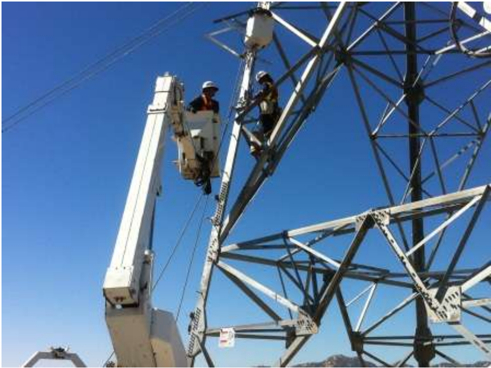
Figure 2: Installing camera equipment at CP100-1. (Link 5)
