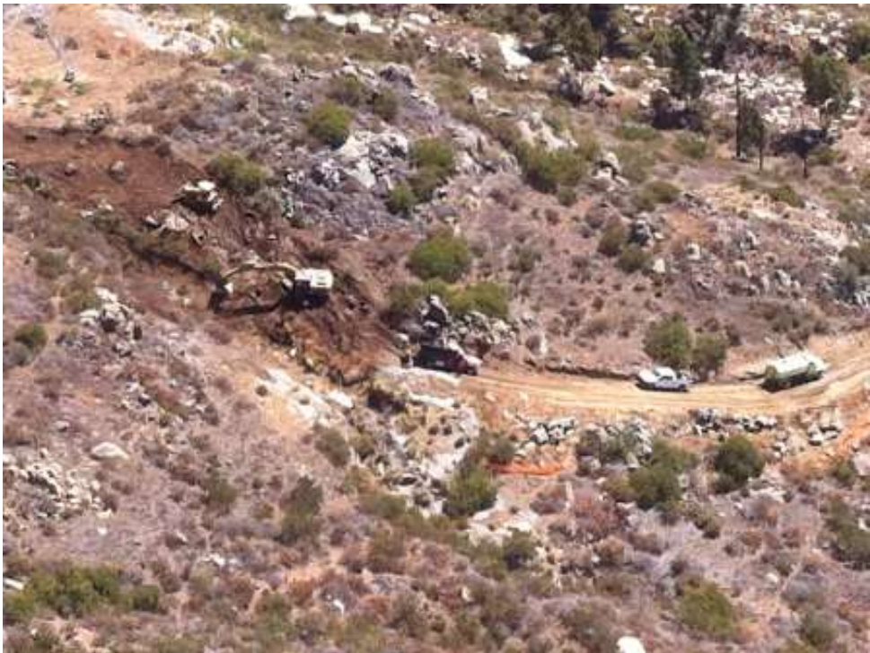
Figure 1: Restoration grading at CP49-1-N. (Link 5)
