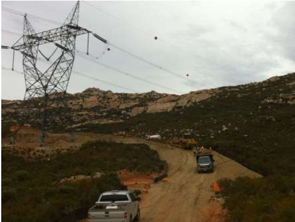
Figure 1: Final grading at EP22-1 pull site. ( Link 2 )
