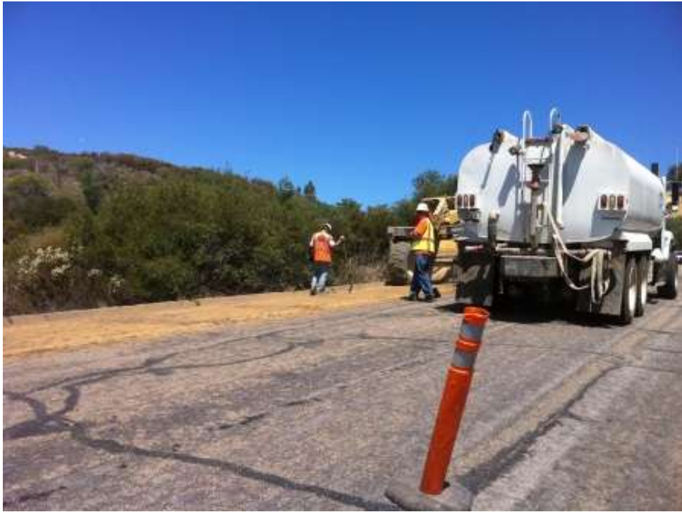
Figure 3: Preparing to pave BBTT. (Link 3)
