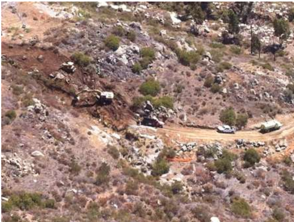
Figure 2: Restoration grading at CP49-1-N. ( Link 5 )
