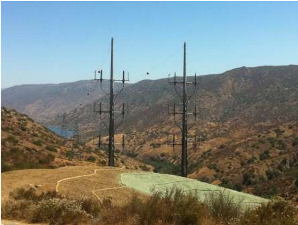
Figure 2: Hydromulching and restoration at CP87/CP88 pull site. (Link 4)
