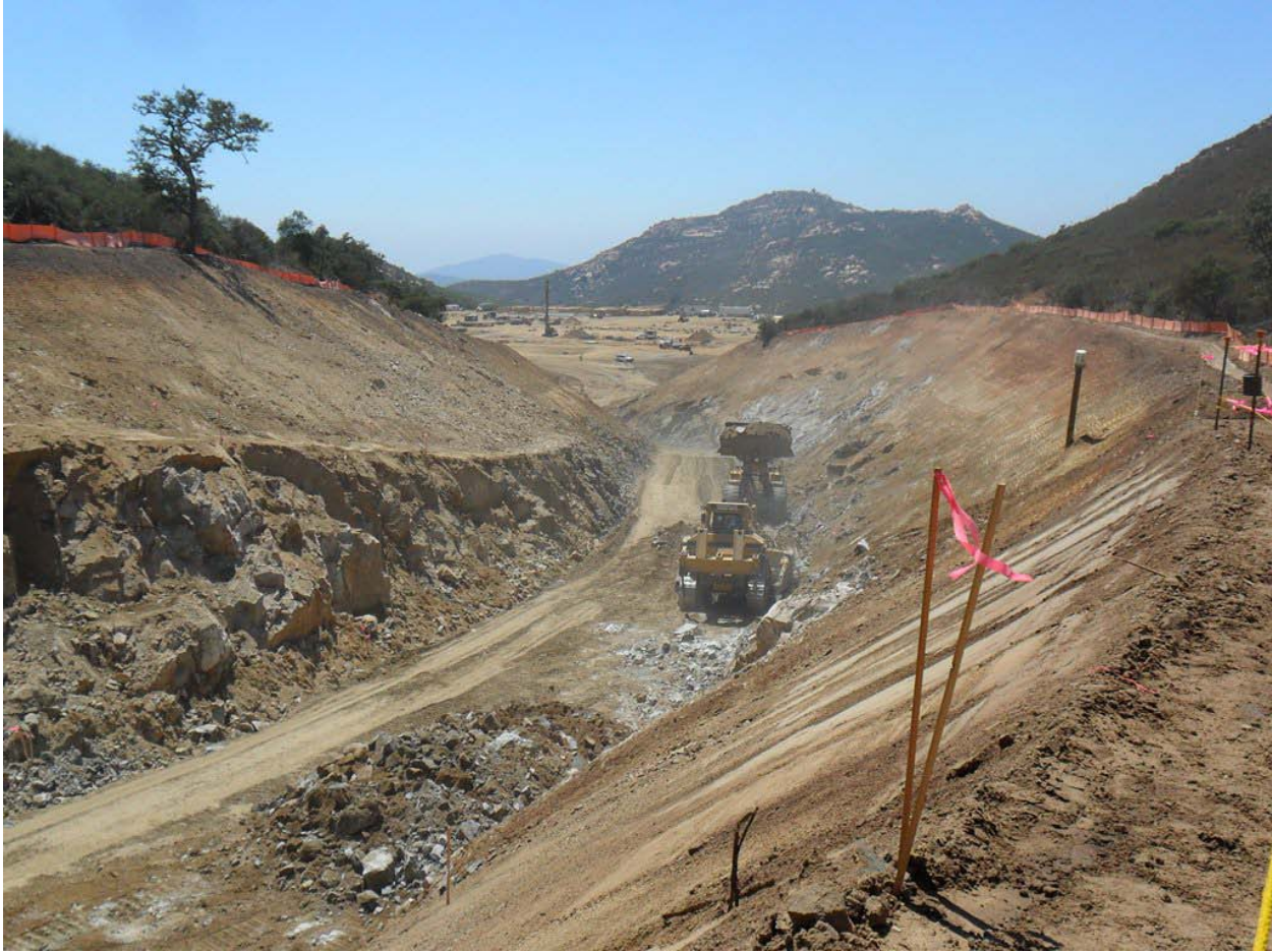
Construction at Suncrest Substation. Photo courtesy of Mark Meridith.
