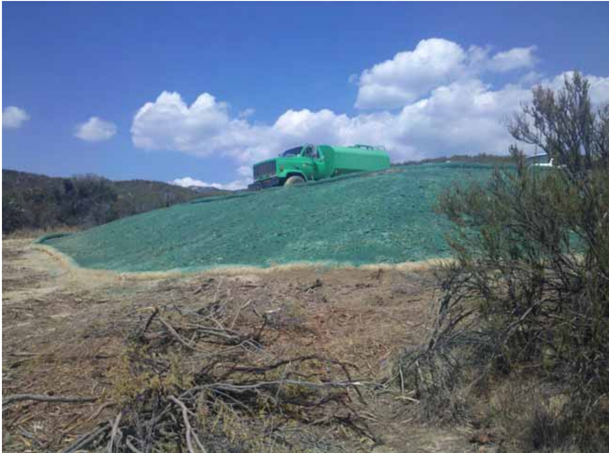
Hydromulch at EP125 pull site. Photo courtesy of Rosina Gallego.
