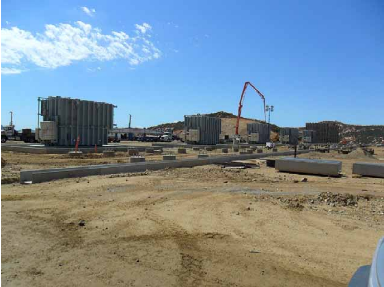
Final transformer delivery to Suncrest Substation. Photo courtesy of Mark Meridith.
