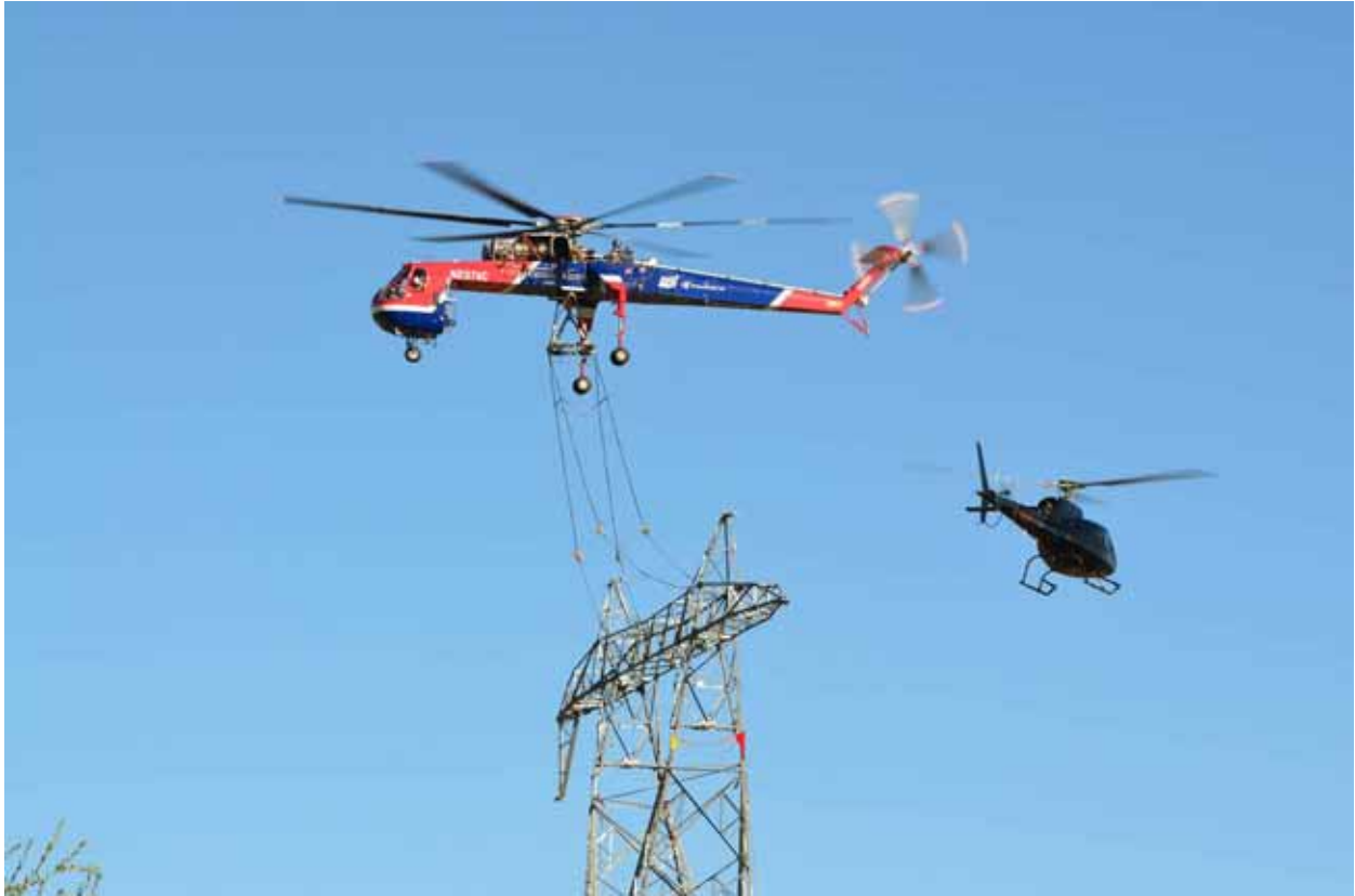
Setting bridge at EP205. Photo courtesy of Rebecca Carson.
