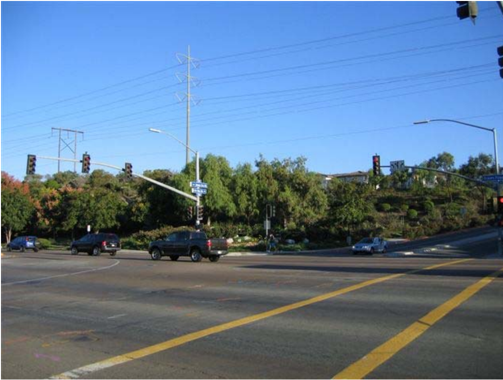
Corner of Ivy Hill Drive and Scripps Poway Parkway (SPP) Proposed 230 kv line would transition from overhead to underground at this point and head west on SPP to I15 where SPP changes name to Mercy Road
