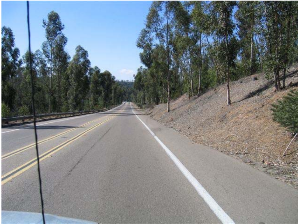
Typical view of Pomerado Road (looking west)
