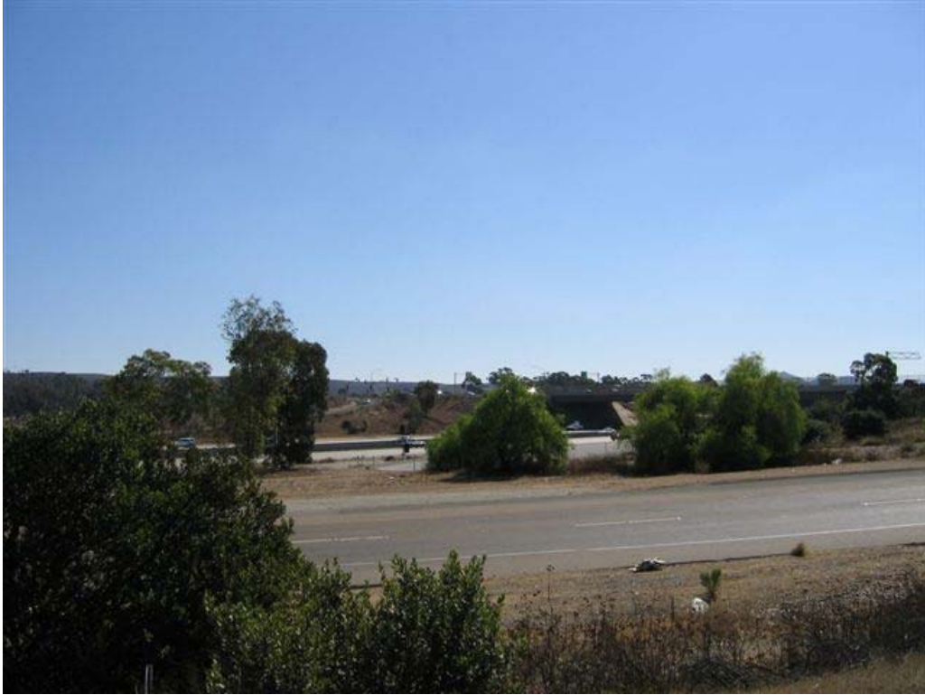
Pomerado Road and Miramar Road overpass at Interstate 15 (looking east).
