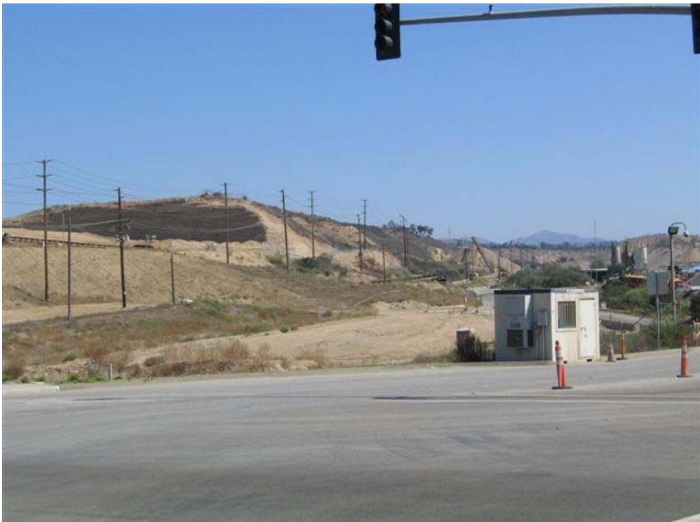
Existing 69 kv lines in Fenton Canyon. View is from Camino Santa Fe looking east.
