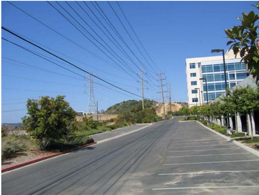
SDG&E North-South ROW east of Interstate 805 looking north
