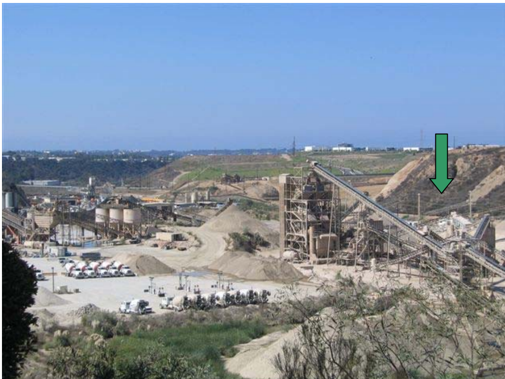
Additional rock quarry operations in Fenton Canyon. Existing 69 kv lines are below green arrow.
