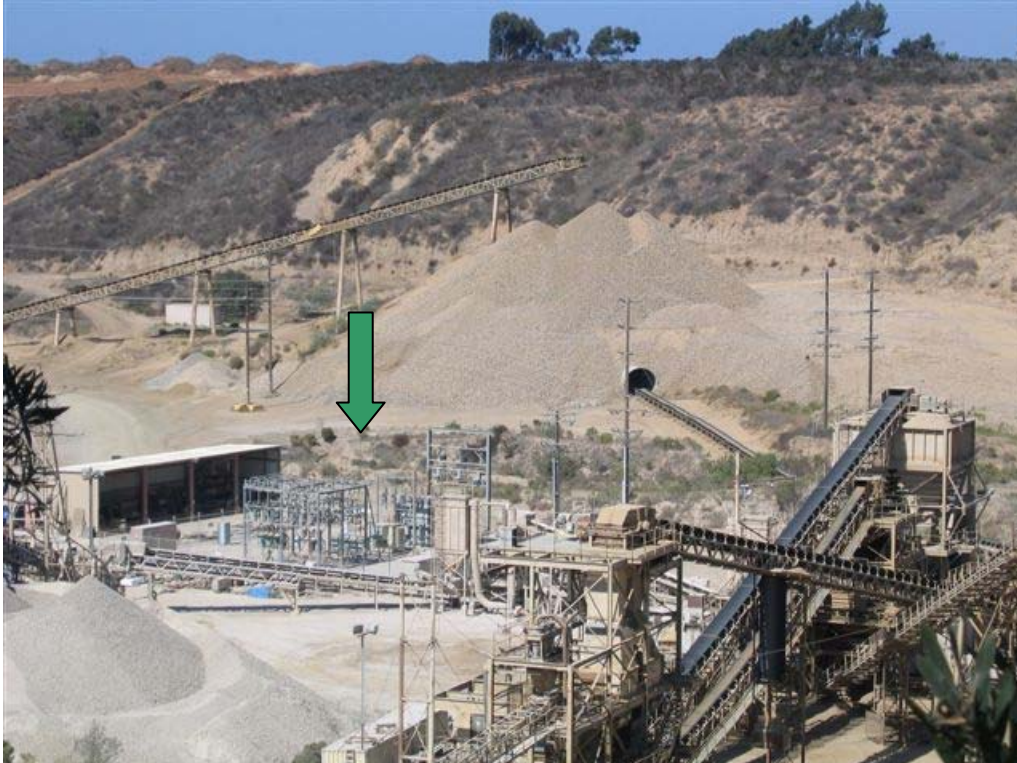
View of rock quarry operation in Fenton Canyon. Fenton substation is below green arrow.
