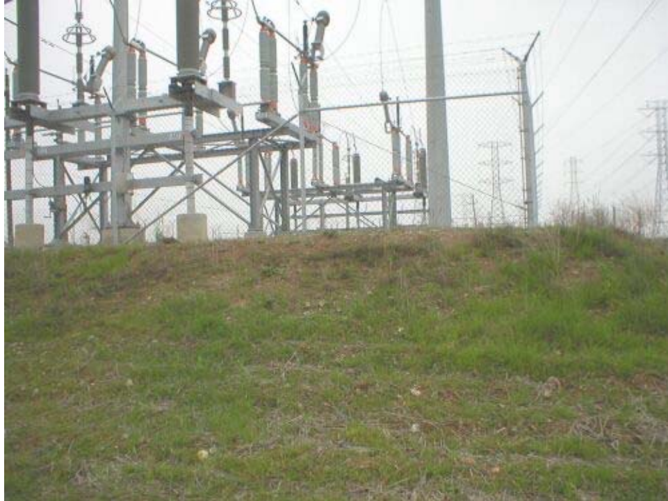
Figure 1 – Transition Station slope area pre-seed application, Phase One.
