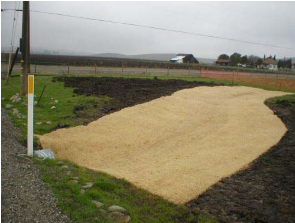
Figure 4 – Added erosion controls within drainage areas along the access road to the Transition Station, Phase Two.
