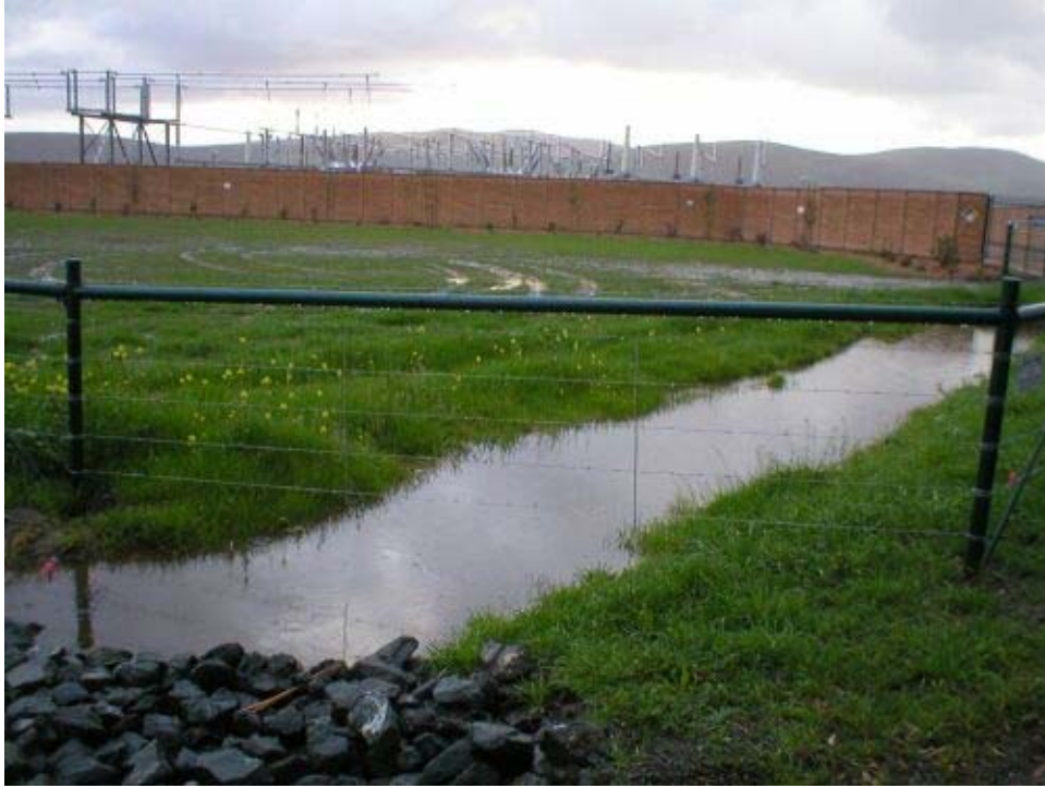
Figure 3 – Flooded drainage at the Cayatano Substation, Phase Two.
