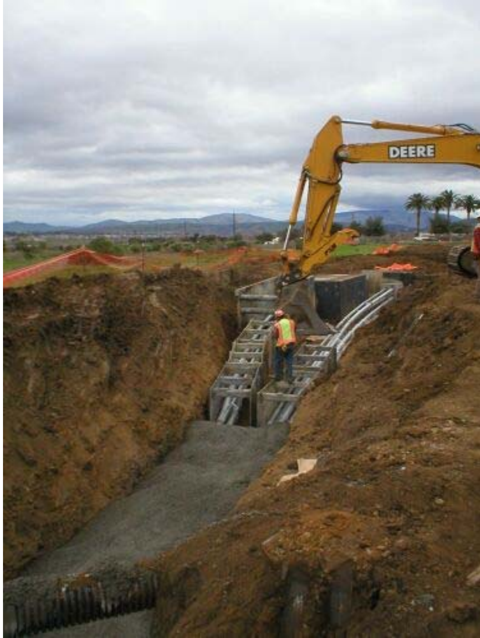
Figure 2 Conduit tie-ins to Vaults 11A and 11B.
