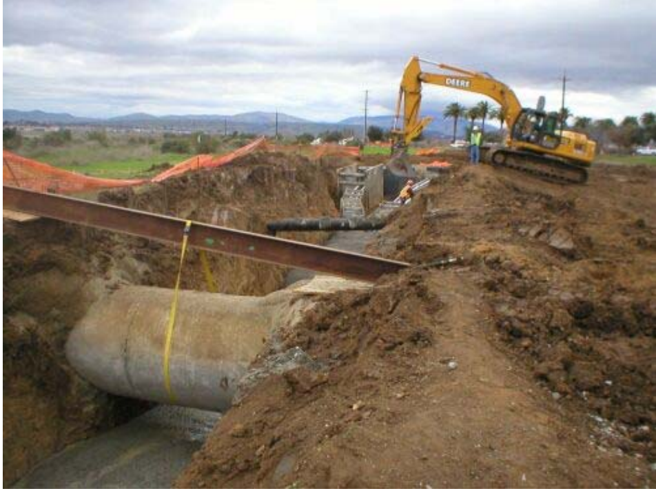
Figure 1 Conduit tie-ins to Vaults 11A and 11B.
