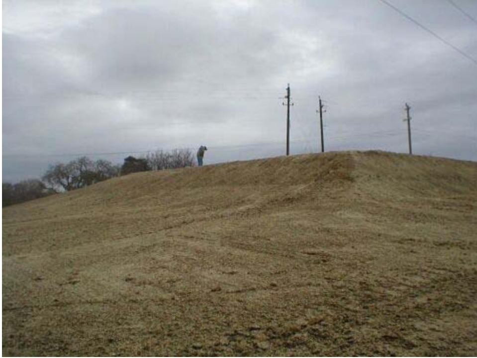
Figure 3 Transition Station pad which was recently hydro-seeded for erosion control purposes.
