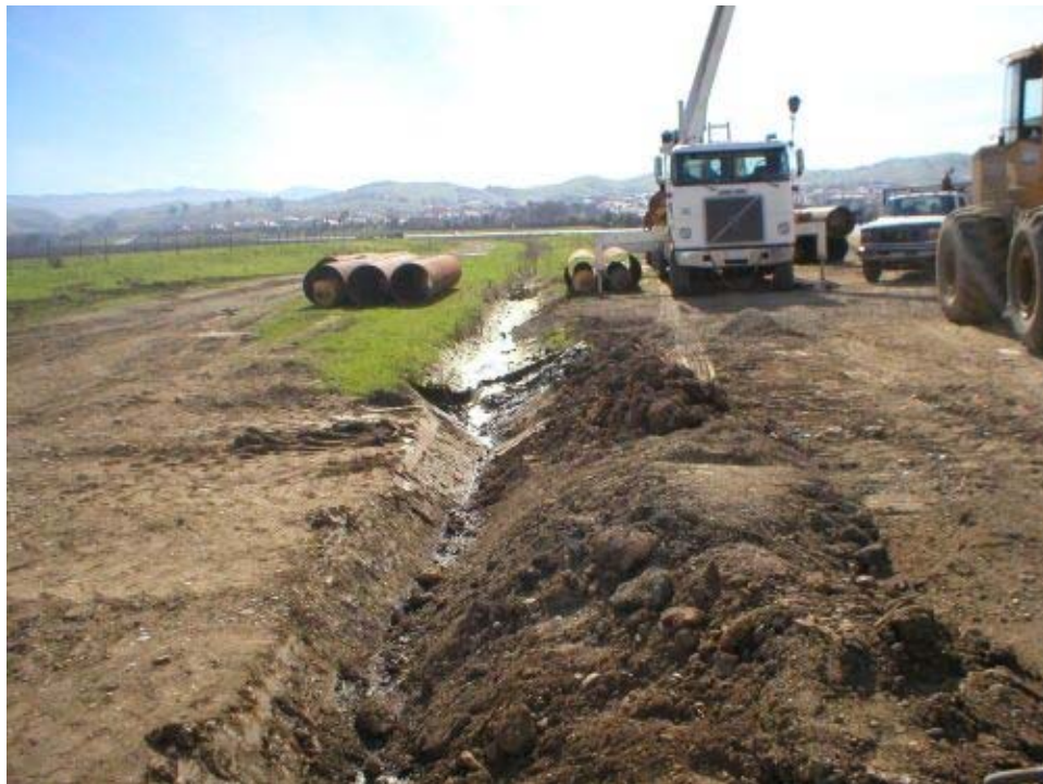
Figure 2 Storm drain near the Isabel Avenue bore.
