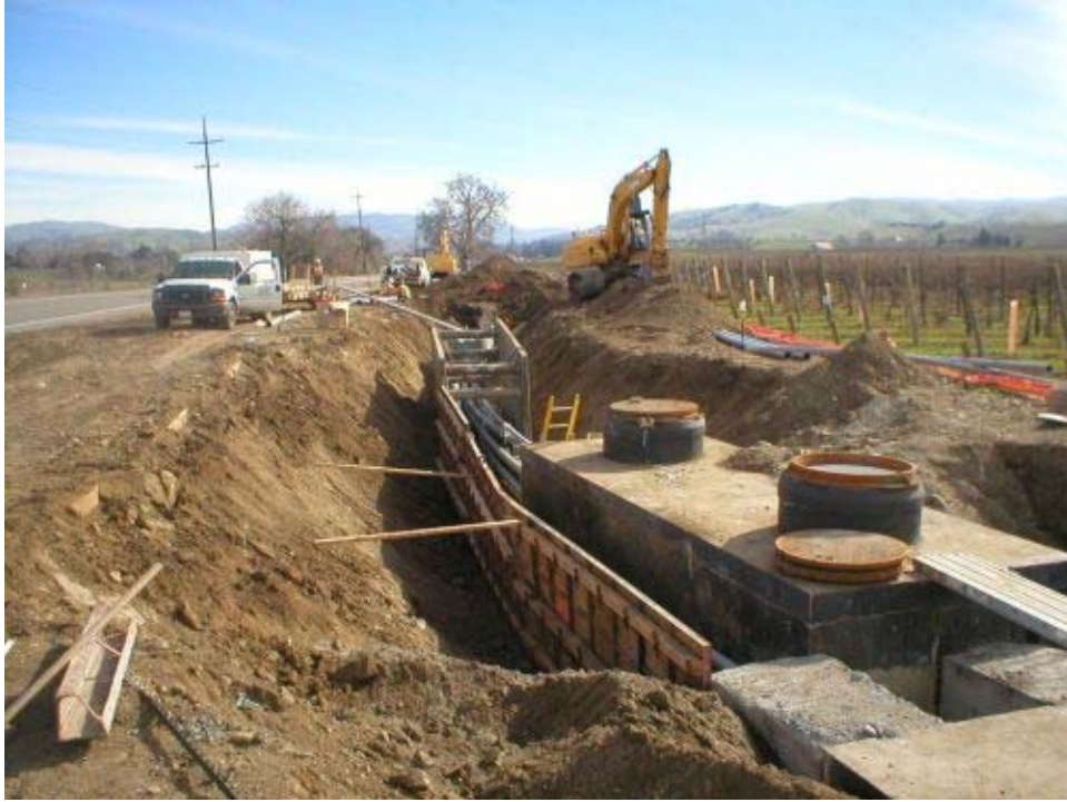
Figure 3 Conduit tie-ins to Vaults 6A and 6B.
