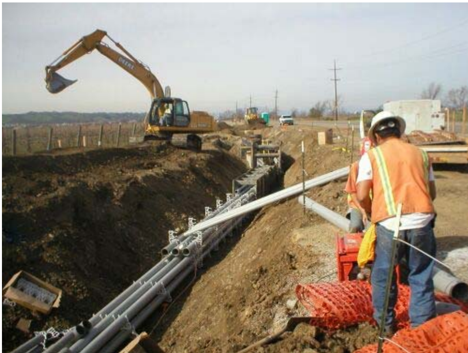
Figure 4 Conduit tie-ins to Vaults 6A and 6B.
