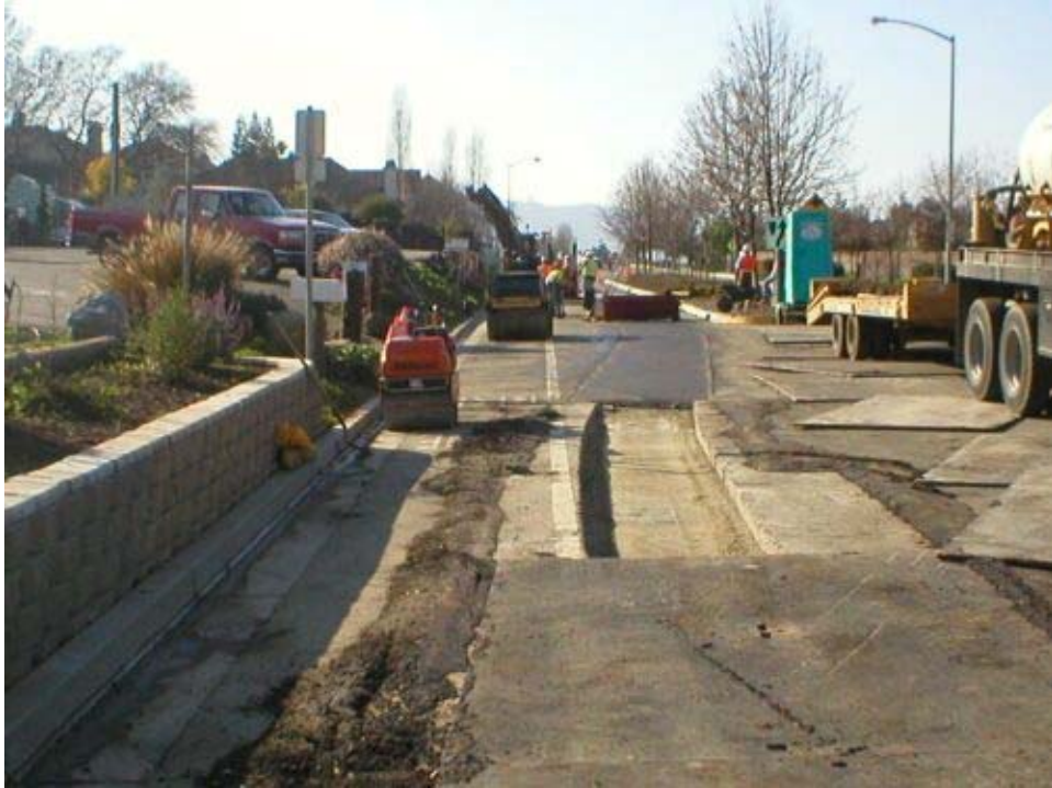
Figure 3 Repavement of trench line along “Old” Vineyard Avenue.
