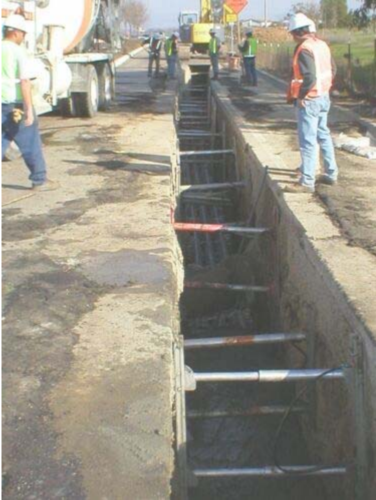
Figure 2 Trench line conduit installation within Vineyard Avenue.
