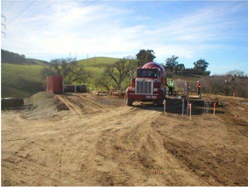
Figure 3 Transition Station foundation work.
