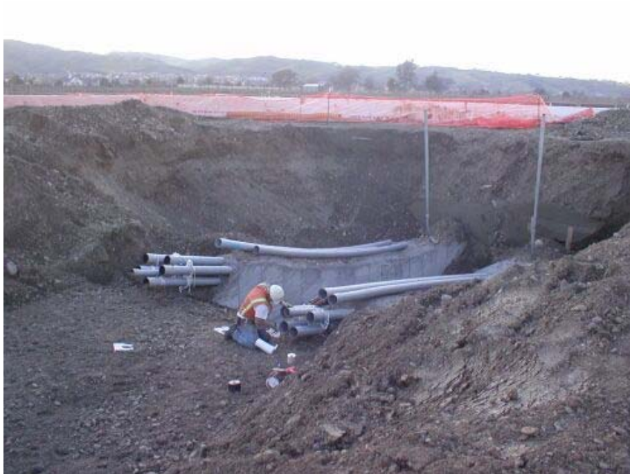
Figure 4 East side of Isabel Avenue bore, tie-in work.
