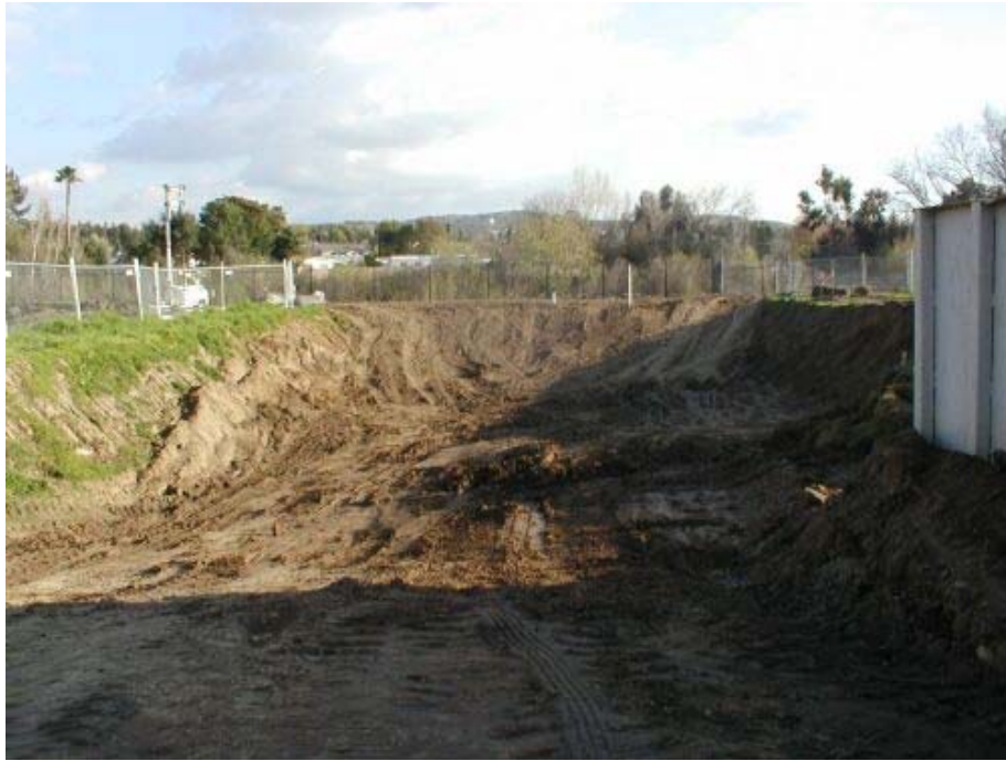
Figure 1 Arroyo del Valle northern bore pit, partially backfilled.
