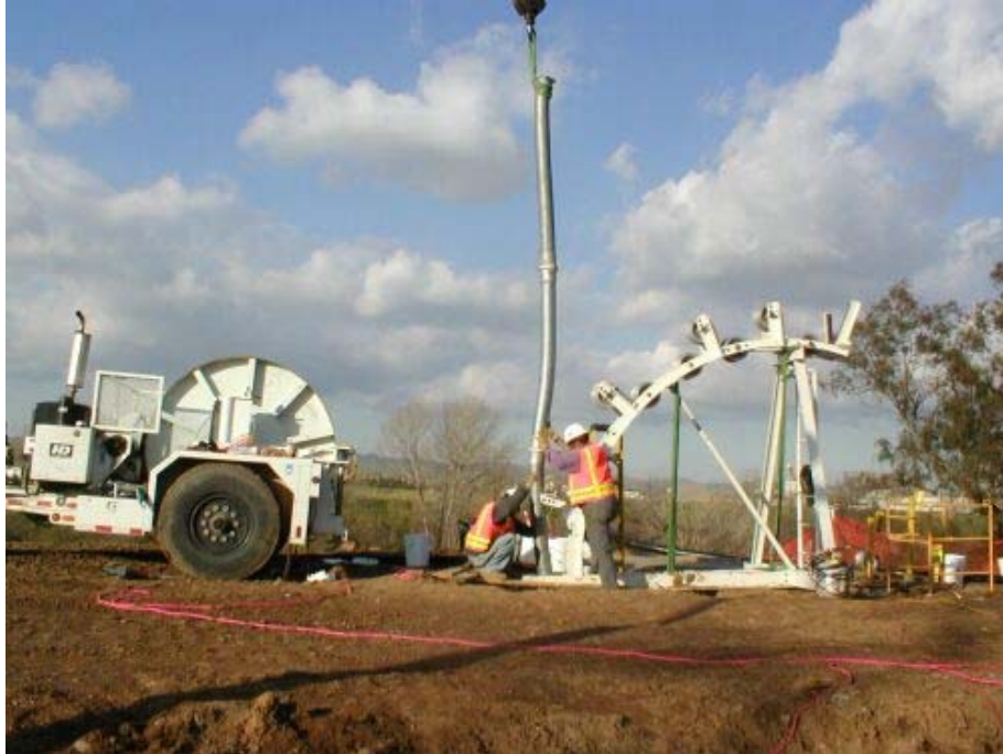
Figure 3 Pulling Cable.
