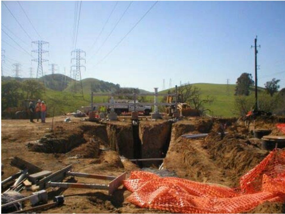
Figure 3 Transition Station line excavation work.
