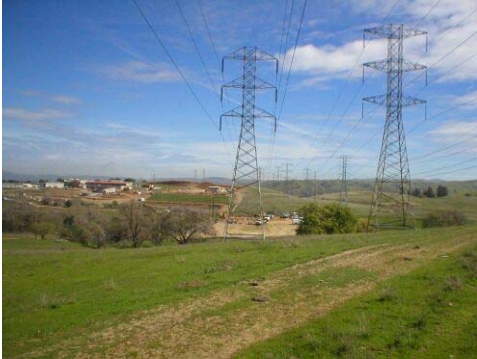
Figure 3 Transition Station viewed from TEWS area. The Boom truck will be placed along the two-track road in the foreground.
