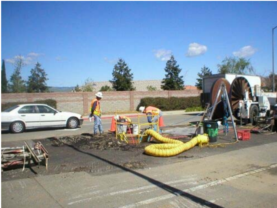
Figure 2 Work at the Vault 17 location along Vineyard Avenue.
