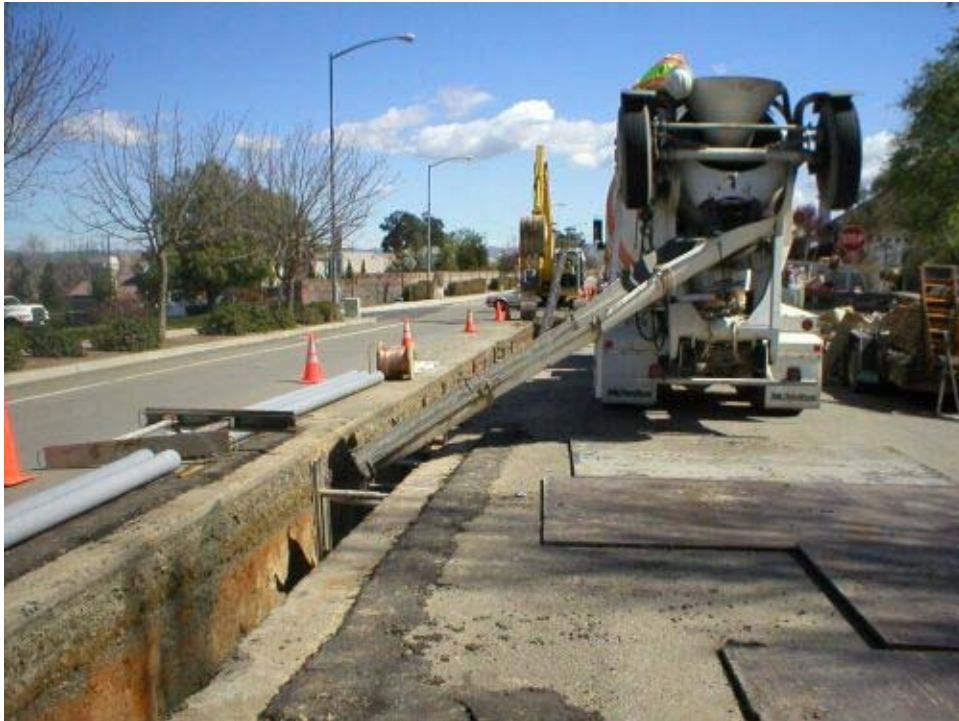
Figure 1 Street trench within Vineyard Avenue between Vault locations 16 and 17.
