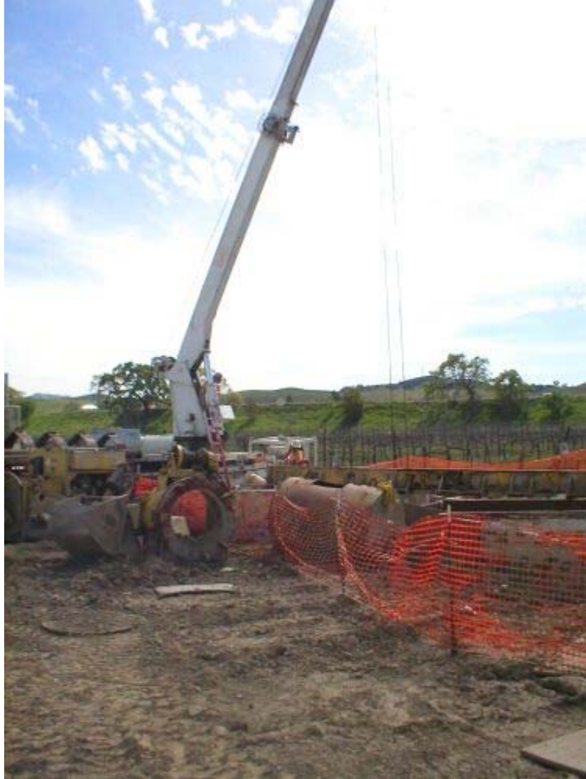
Figure 1 Highway 84 boring operations.
