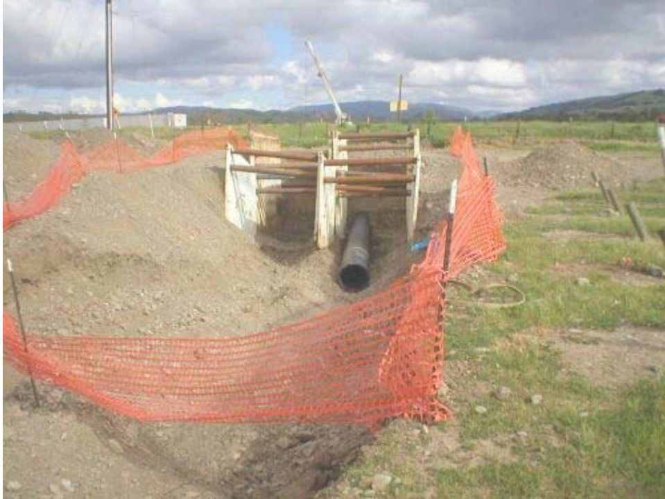
Figure 4 The first of the two bores under Highway 84 has been completed.
