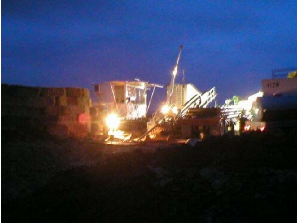
Figure 2 - New Vineyard Road Tributary Bore Rig Lighting
