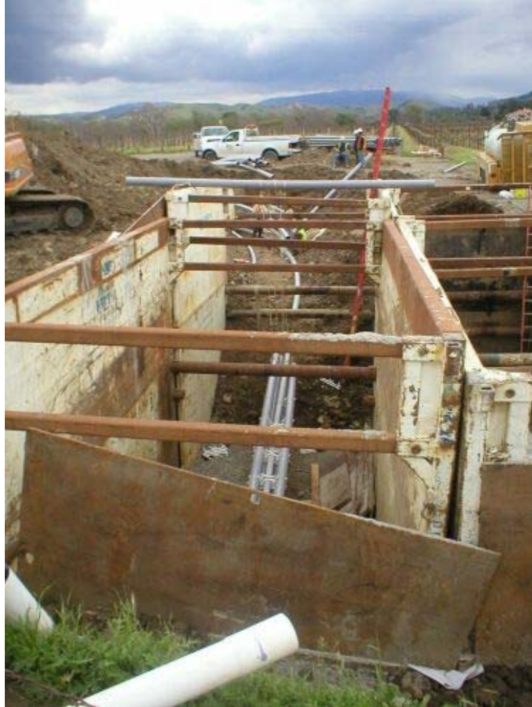
Figure 4 - Highway 84 bore tie-in work
