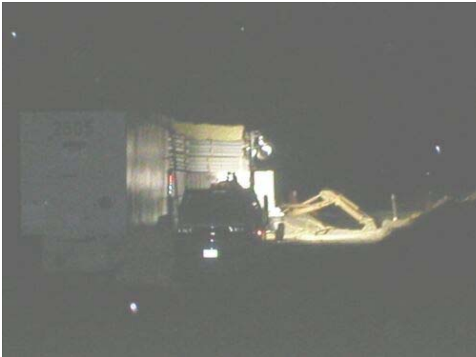
Figure 3 - New Vineyard Road Tributary Bore Exit Pit Lighting.
