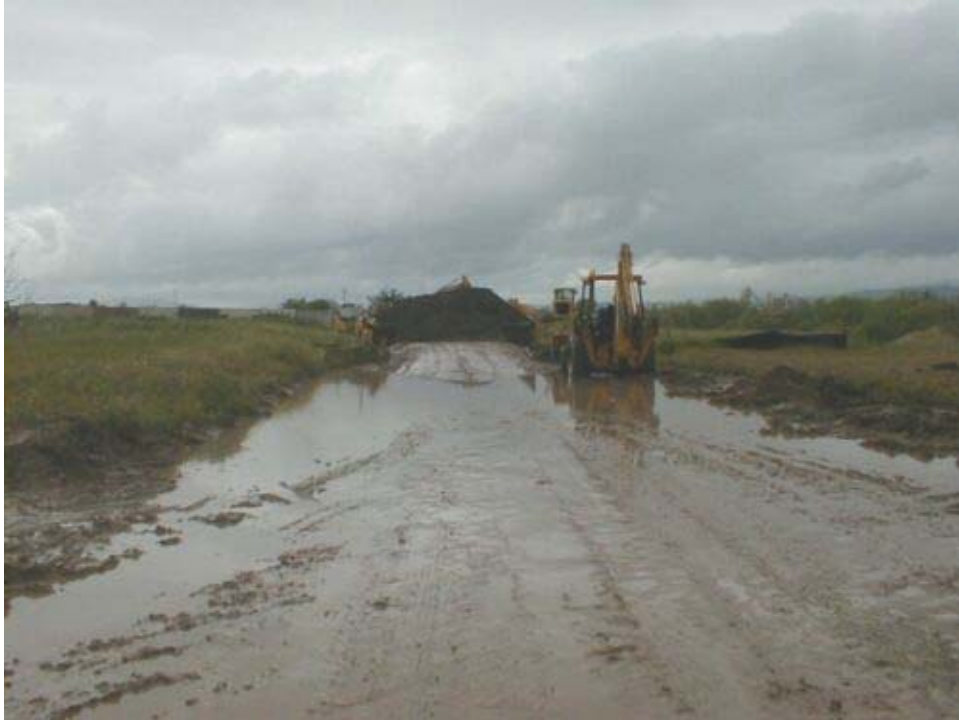
Figure 2 - New Vineyard Road Tributary tie-in work.
