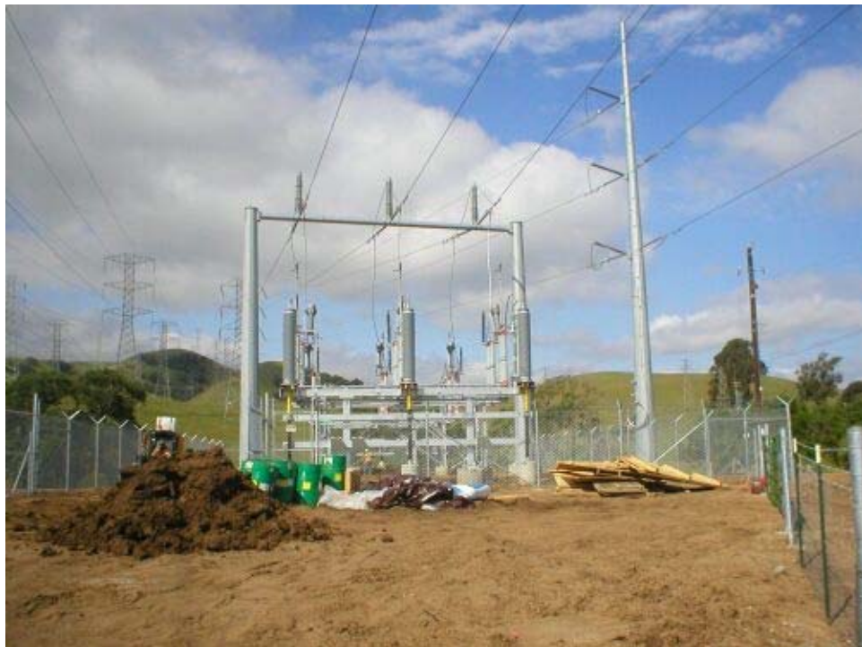
Figure 3 – Clean-up and grading activities at the Transition Station.
