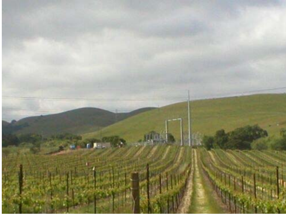
Figure 2 – Far view of the Transition Station.
