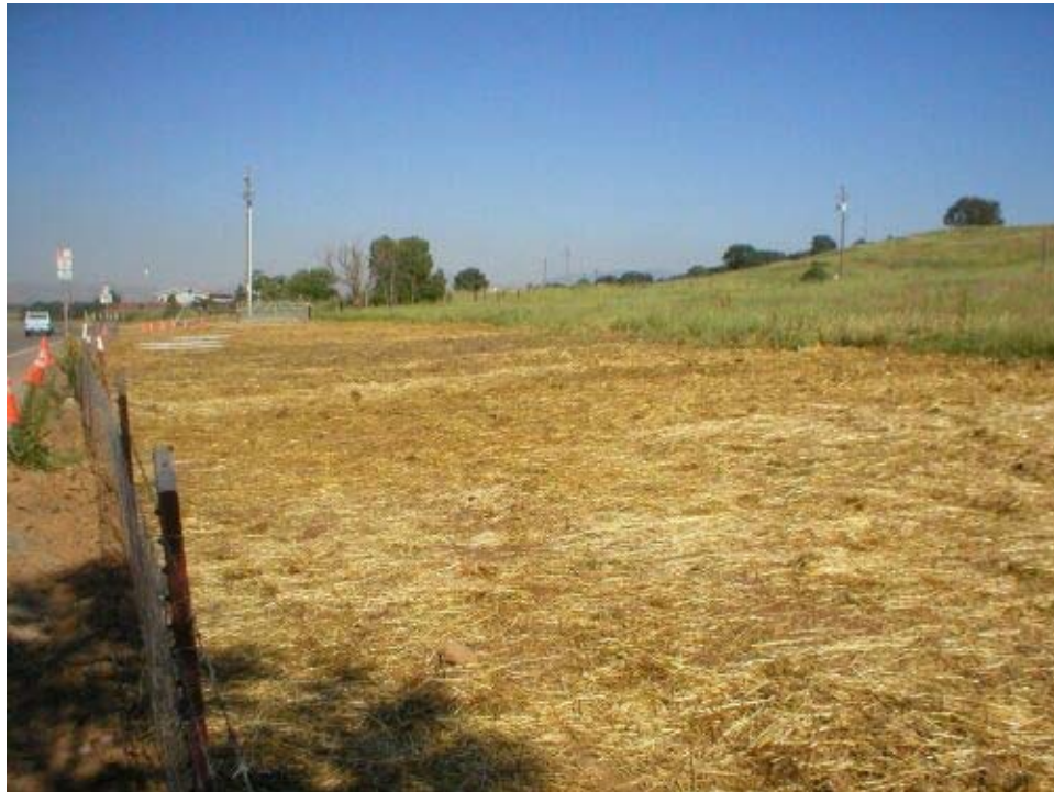
Figure 1 – Mulch cover applied for erosion control approaching the Vault 15 area.
