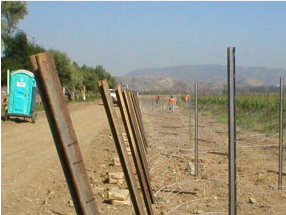
Figure 2 – Vine row replacement work along “Old” Vineyard Avenue.
