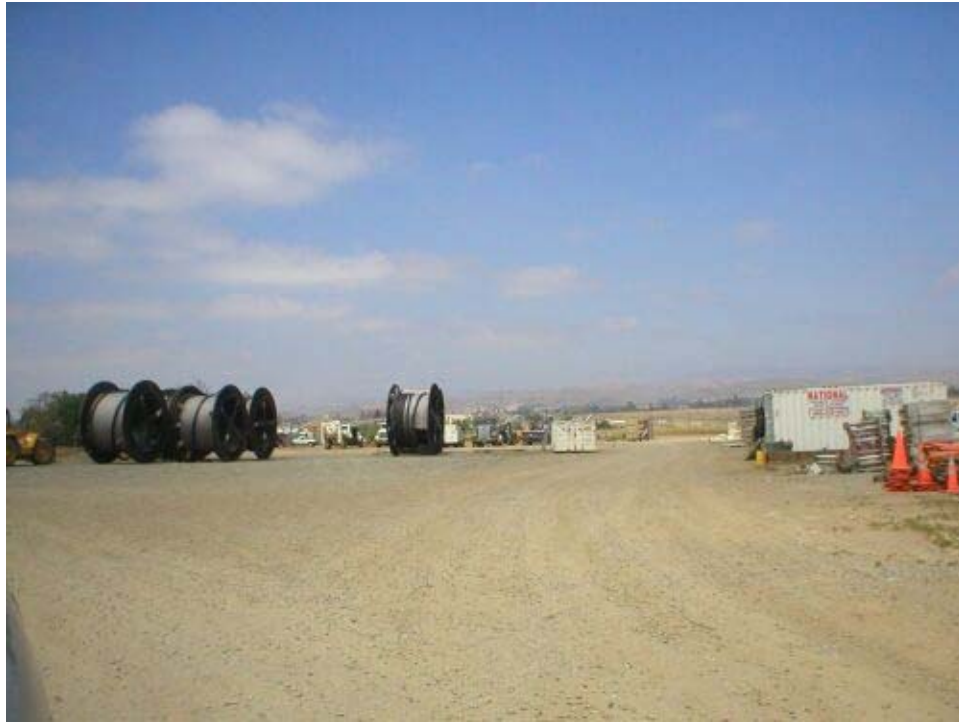
Figure 1 – Mueller lay down yard, Phase One.
