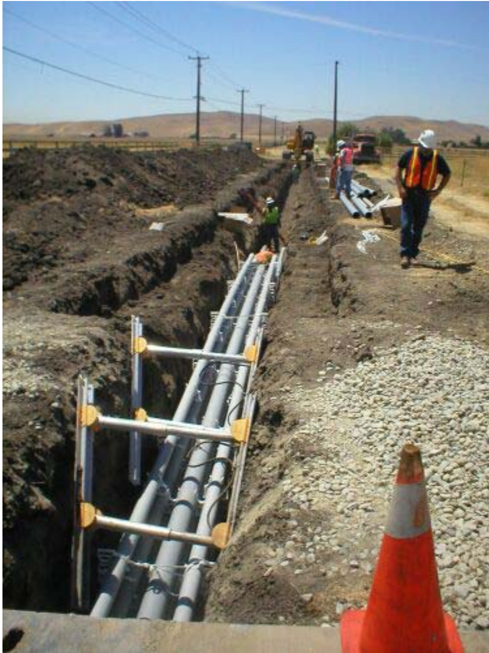
Figure 2 – Trenching and conduit installation along May School Road, Phase Two.
