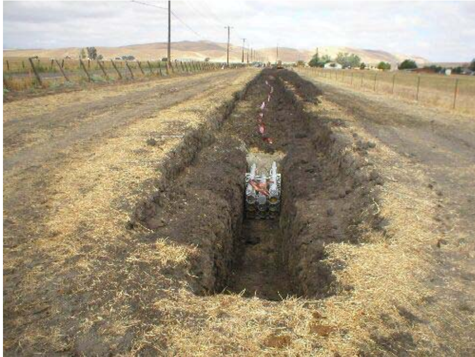
Figure 1 – Trenching and conduit installation along May School Road, Phase Two.
