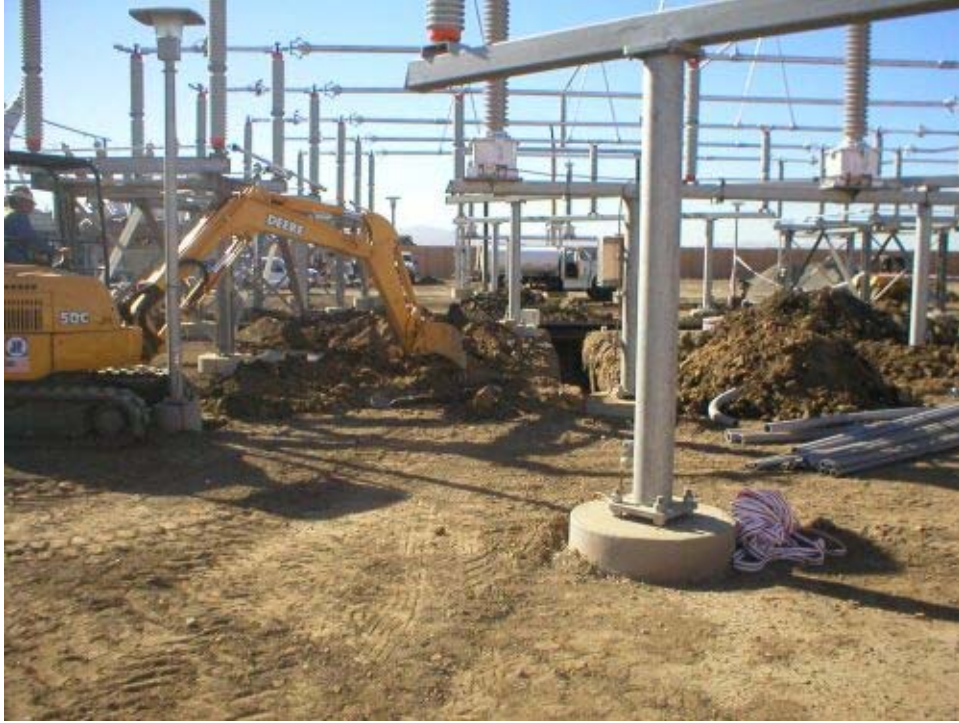
Figure 1 – Trenching at the Cayetano Substation, Phase Two.
