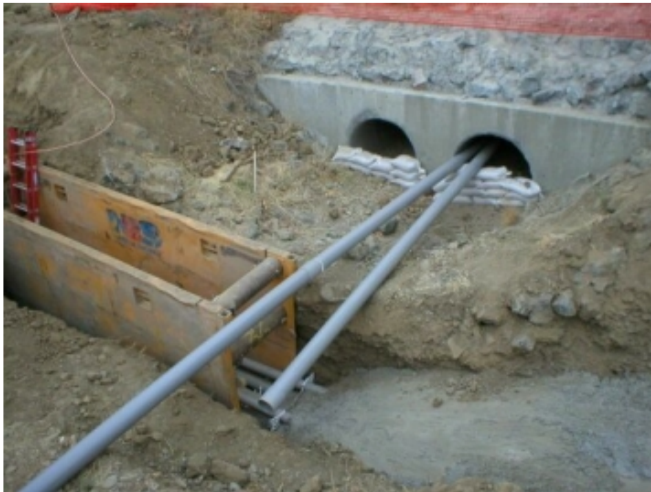
Figure 2 Sediment control devices and culvert at the dry drainage at Station 160+00.
