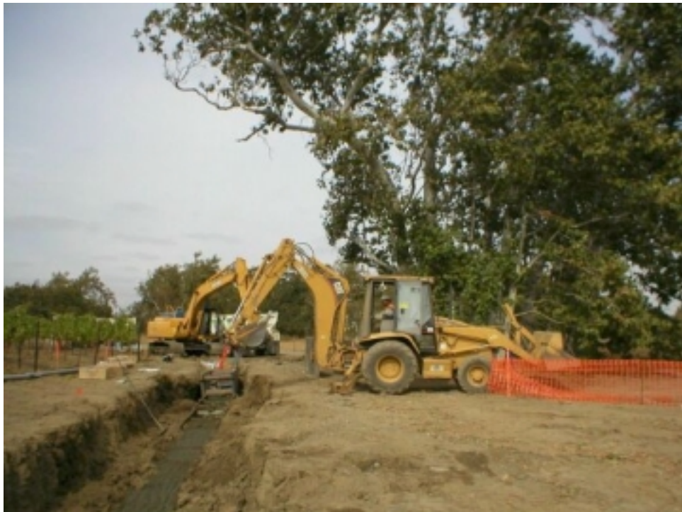
Figure 4 Exclusion fence removal at Sycamore heritage trees.
