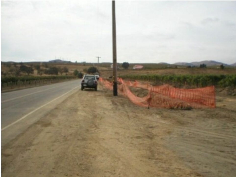
Figure 3 Open trench line adjacent to Zone 7 Access Road.
