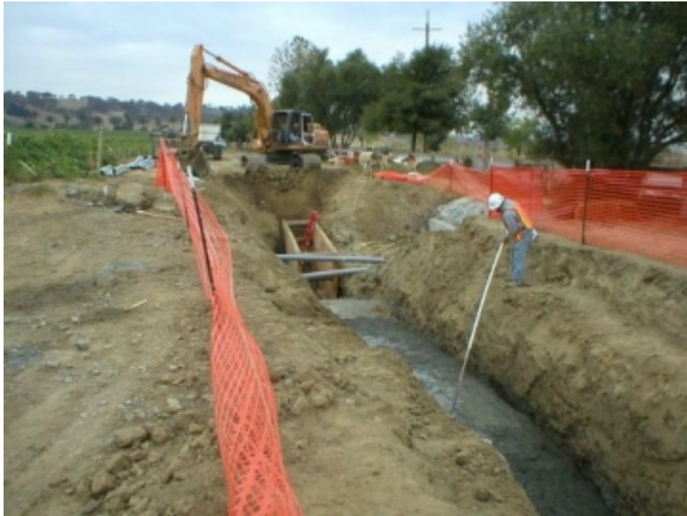
Figure 1 Trenching and conduit installation at the dry drainage at Station 160+00.
