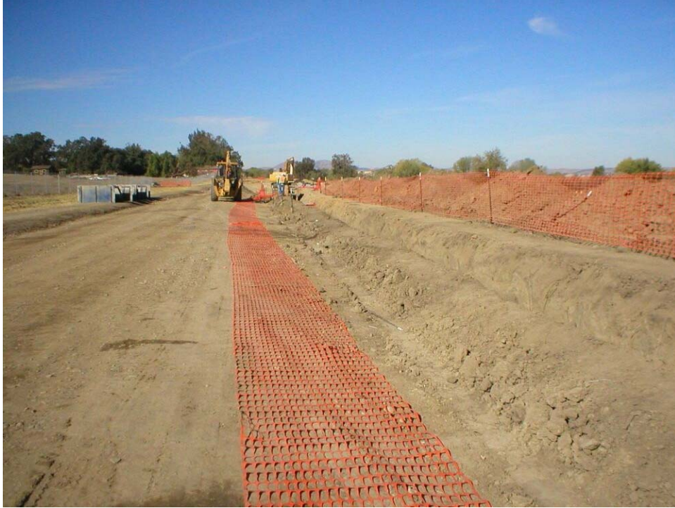
Figure 1 Trenching and conduit installation along New Vineyard Road.
