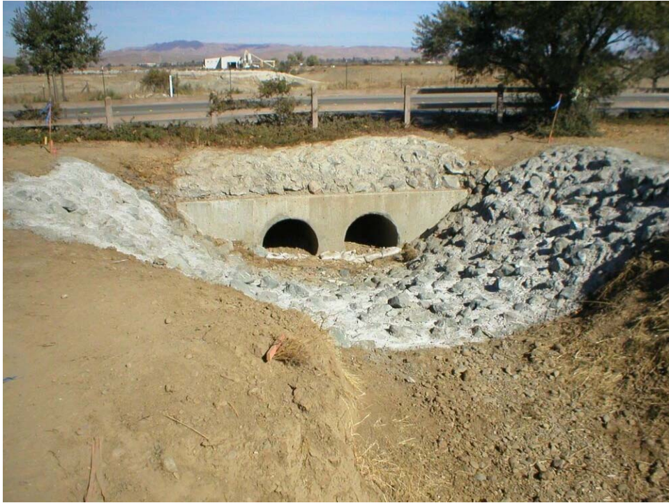
Figure 2 Post installation restoration at the dry drainage at Station 160+00.
