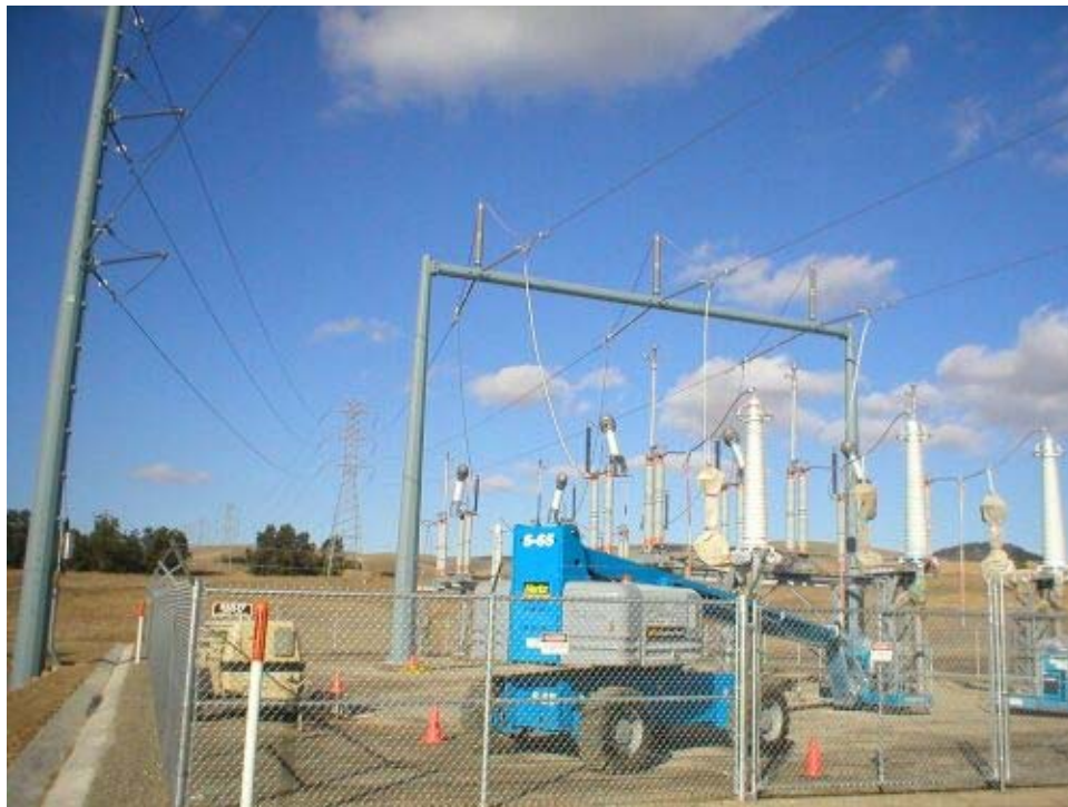
Figure 4 – Transition Station chain link fence, Phase Two.
