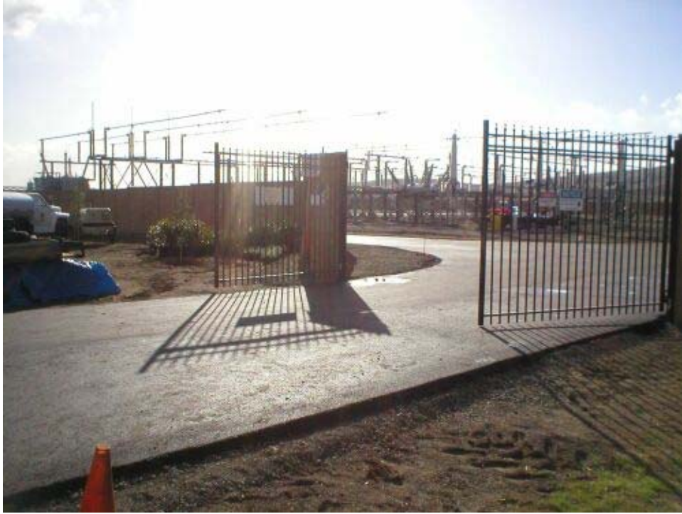
Figure 1 – Asphalt driveway and paving at the Cayetano Substation, Phase Two.
