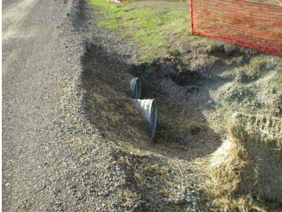
Figure 3 – Culvert along the access road to the Transition Station, Phase Two.
