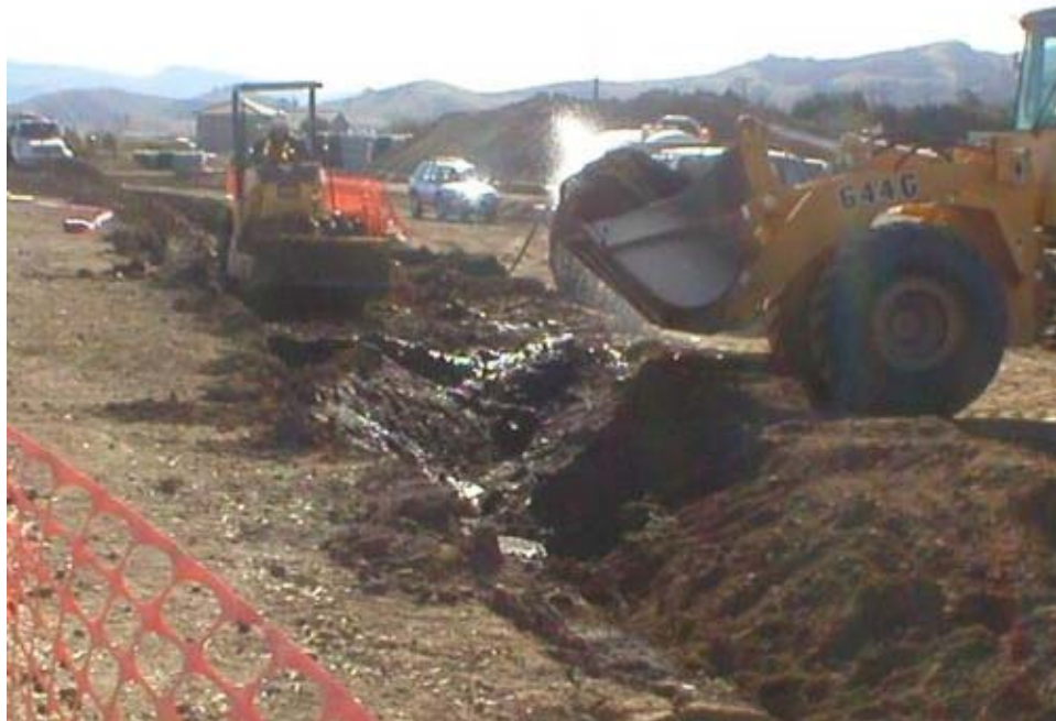
Figure 1 The backfill of trench line along New Vineyard Road.
