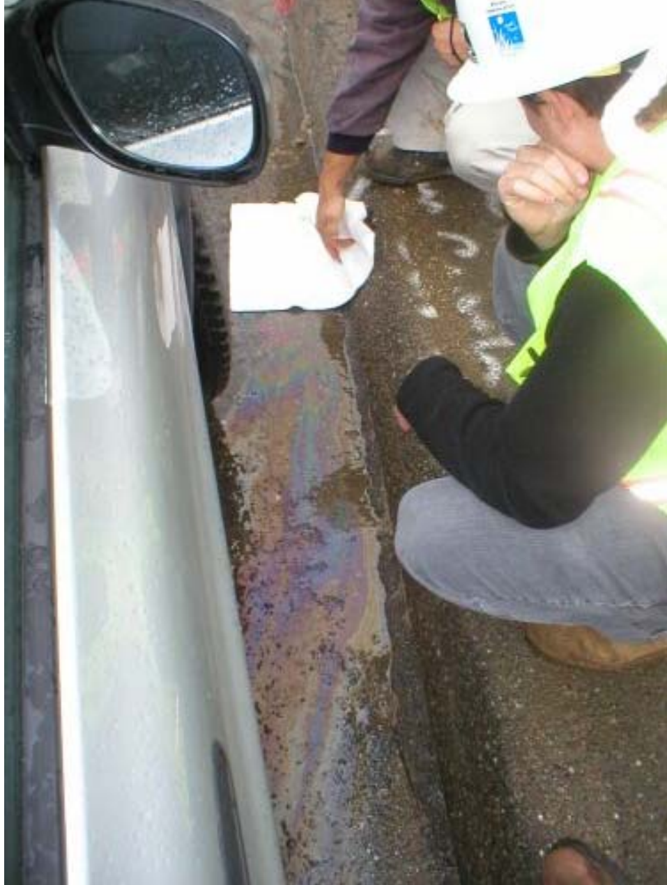
Figure 1 Petroleum clean-up near a storm drain adjacent the Arroyo northern bore pit.
