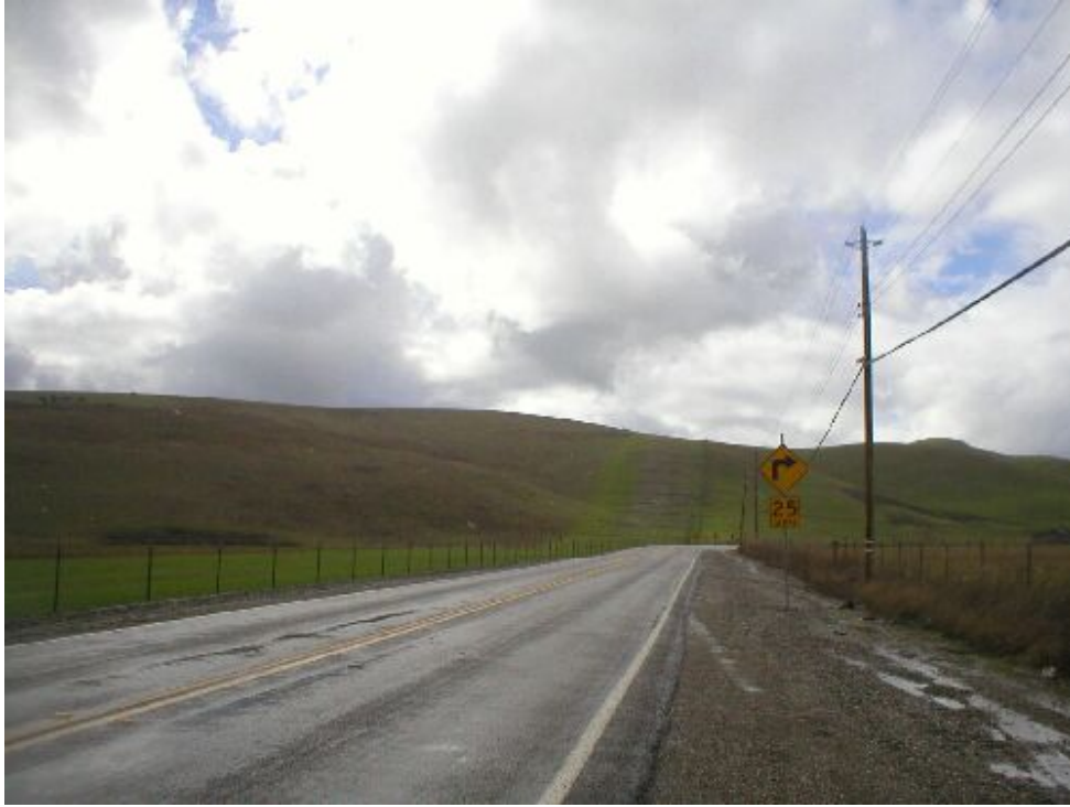
Figure 1 – View of the underground alignment along a steep slope extending from Manning Road off North Livermore Ave. – February 28, 2006.
