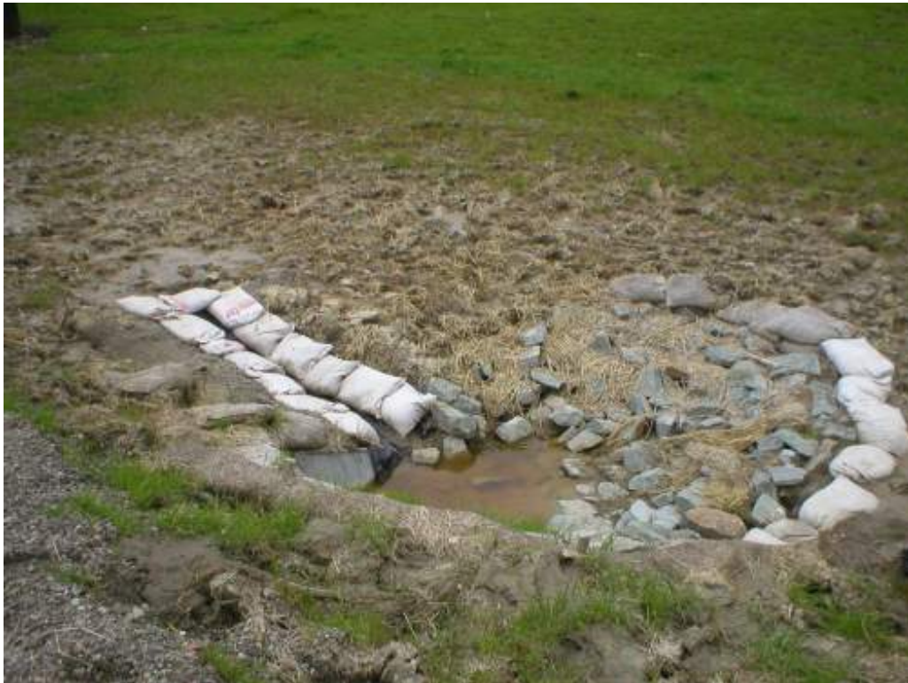
Figure 2 – Opus and NVC repaired culvert inlet area along Moller Road, March 30, 2006.
