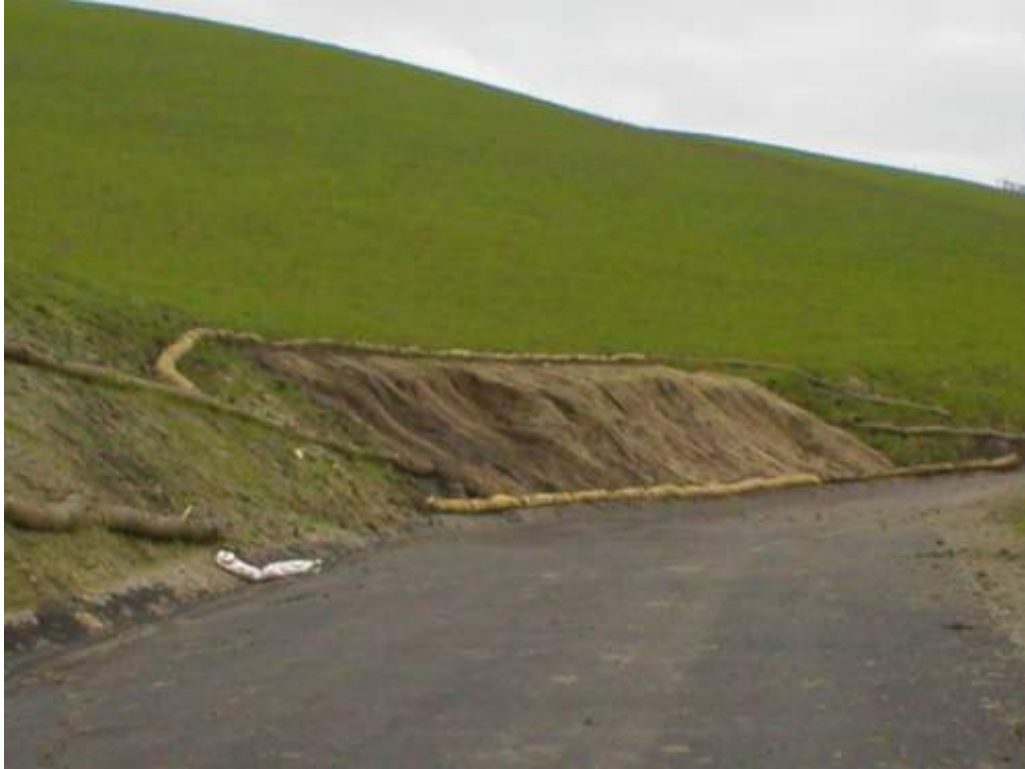
Figure 1 – NVC crews removed loose soil and installed jute netting and wattles along the landslide area along Road 6, March 30, 2006.
