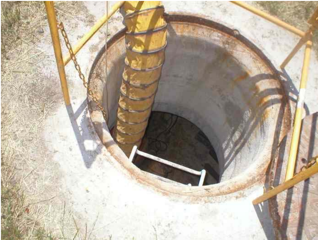
Figure 2 – Jenson PreCast working at Vault 1, June 6, 2006.
