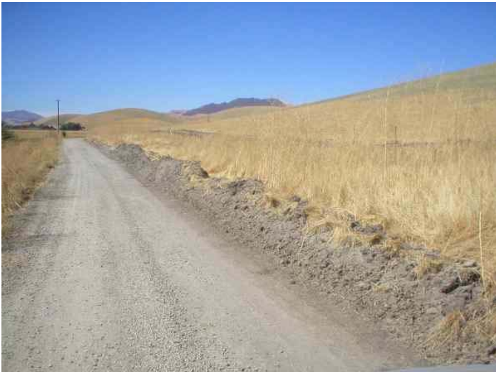
Figure 2 – Road five after re-grading was conducted. July 11, 2006.
