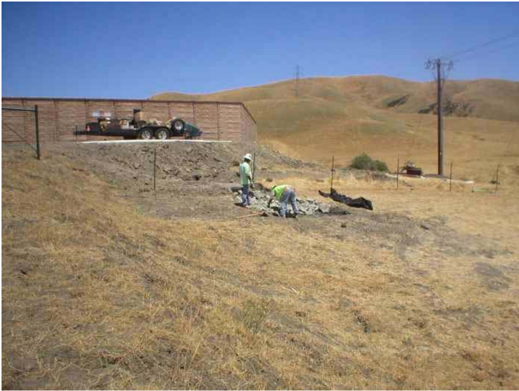
Figure 3 – Vitale & Sons installing irrigation line around the North Dublin Substation. July 7, 2006.
