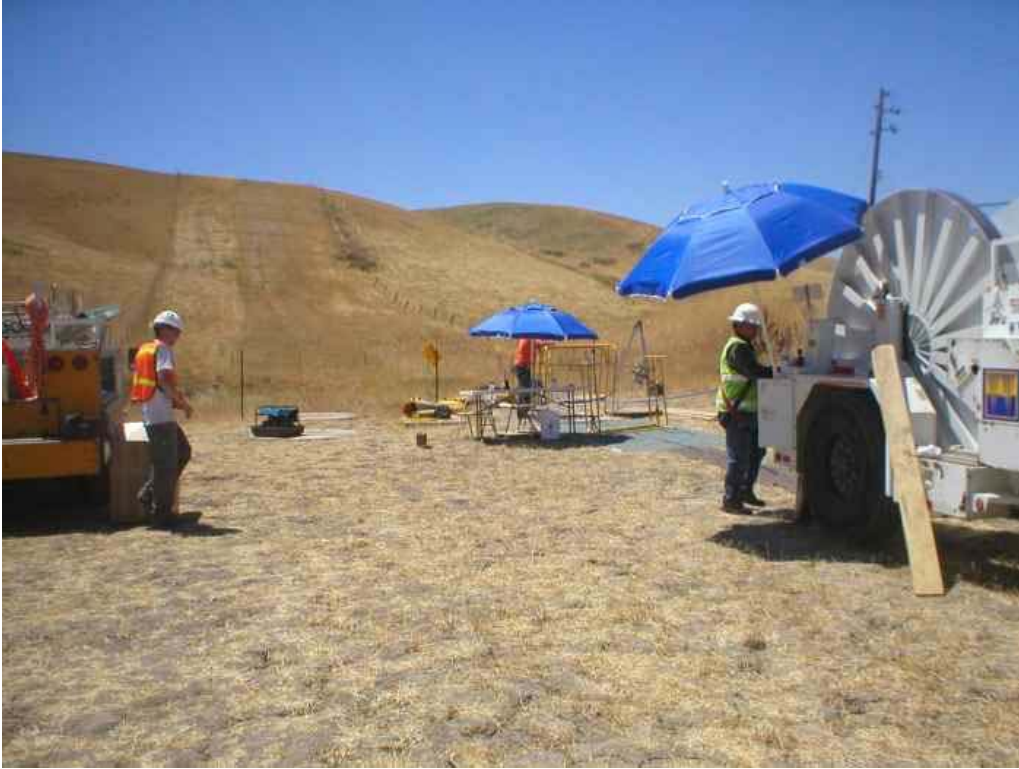
Figure 1 – Cable pulling activities at Vault 5. July 7, 2006.
