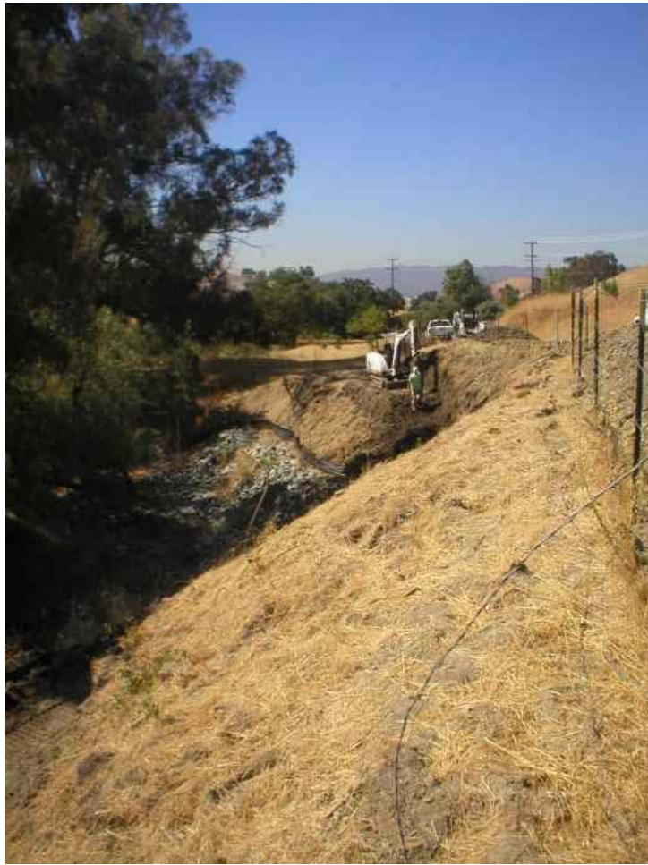
Figure 3 – Bank stabilization work adjacent to Tassajara Creek, August 10, 2006.
