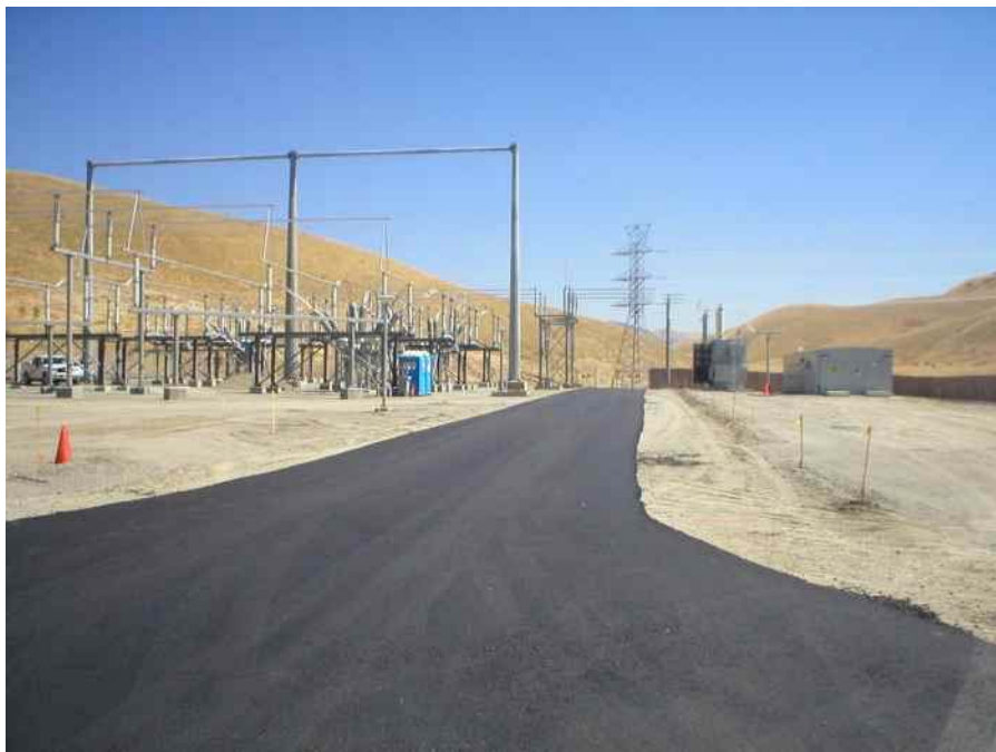
Figure 5 – Granite laid asphalt at the North Dublin Substation, August 10, 2006.
