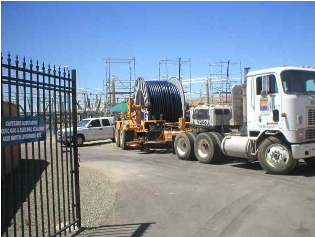
Figure 1 – At the Cayetano Substation, cable was pulled through Vault 2. August 10, 2006.
