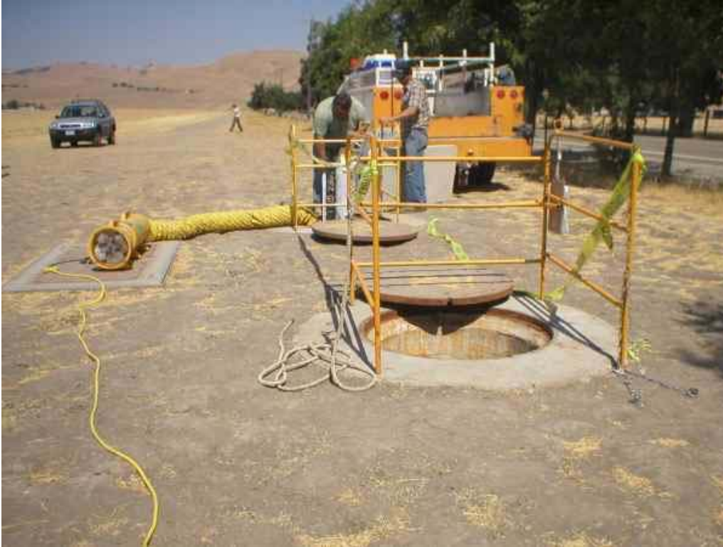
Figure 1 – Wilson crews cleaned and stenciled inside of vaults, September 13, 2006.
