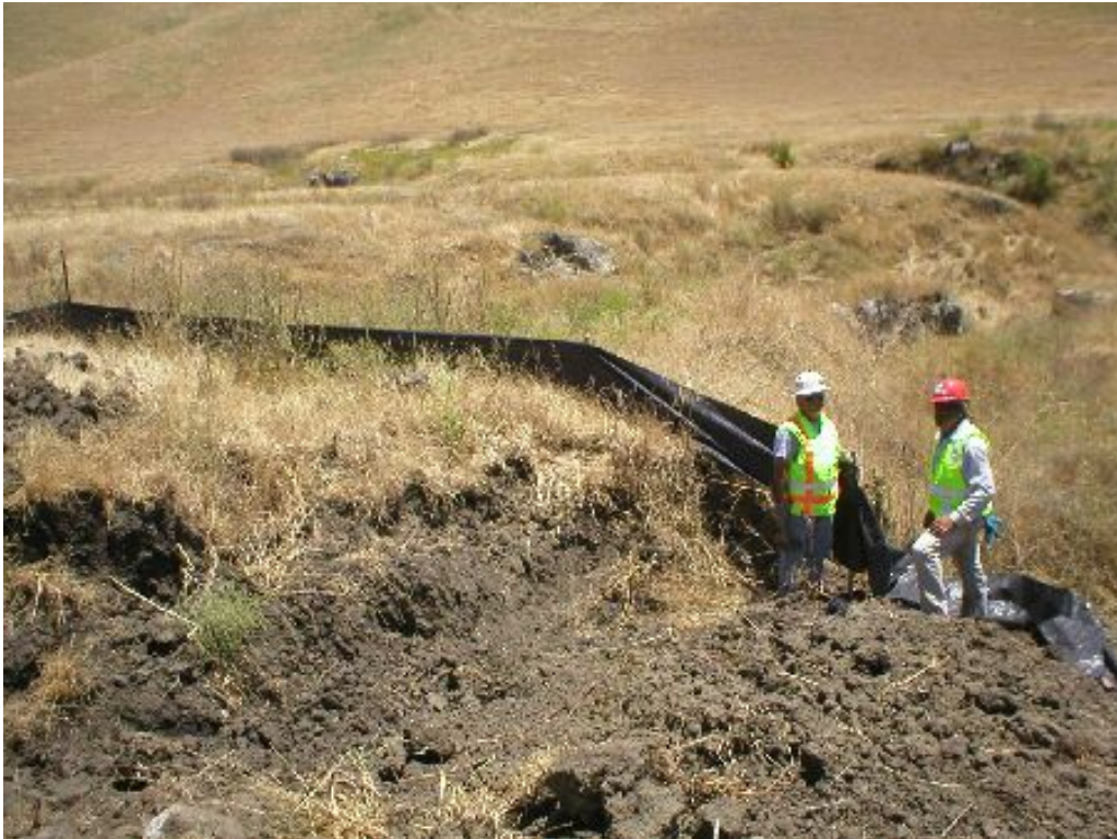
Figure 6 – Moller access road sediment fence installation, Phase Three.
