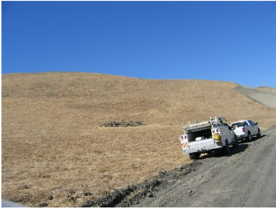
Figure 5 – Tower 1 construction, August 31, 2005.
