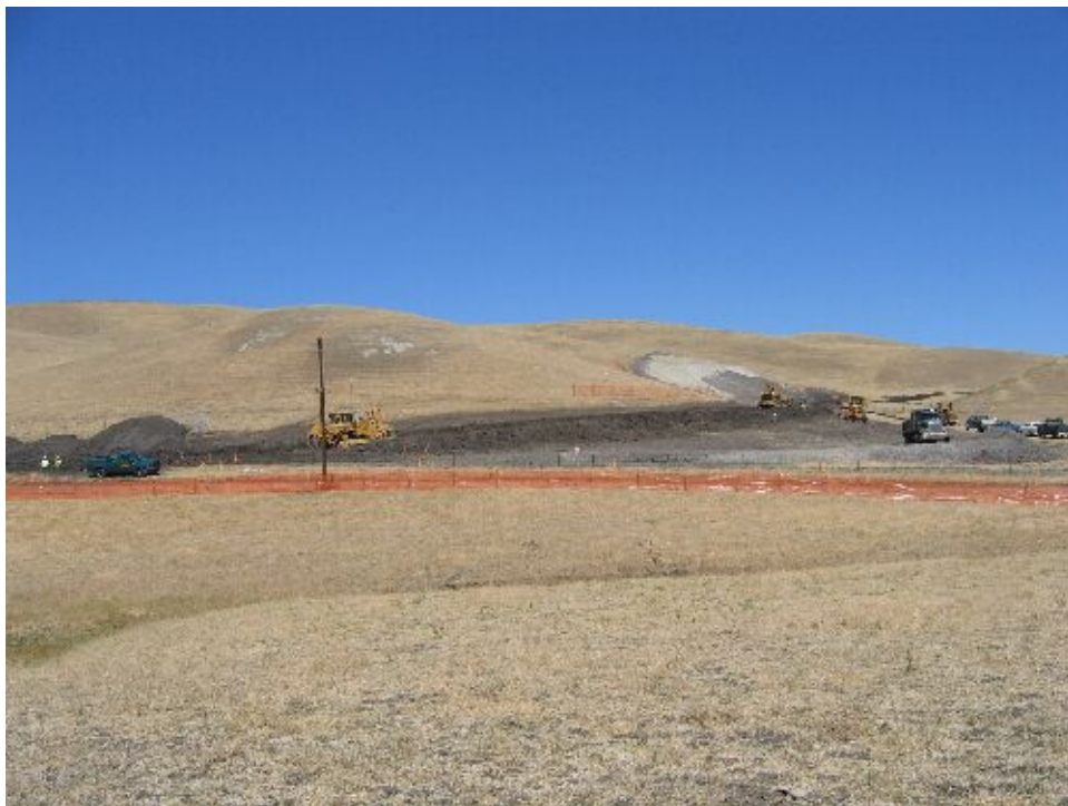
Figure 2 – Granite construction along Road 7, August 31, 2005.
