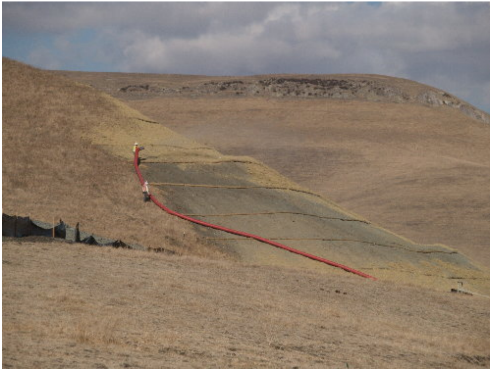
Figure 3 – Crew spreading straw over slopes after hydroseeding along Moller Ranch Road.
