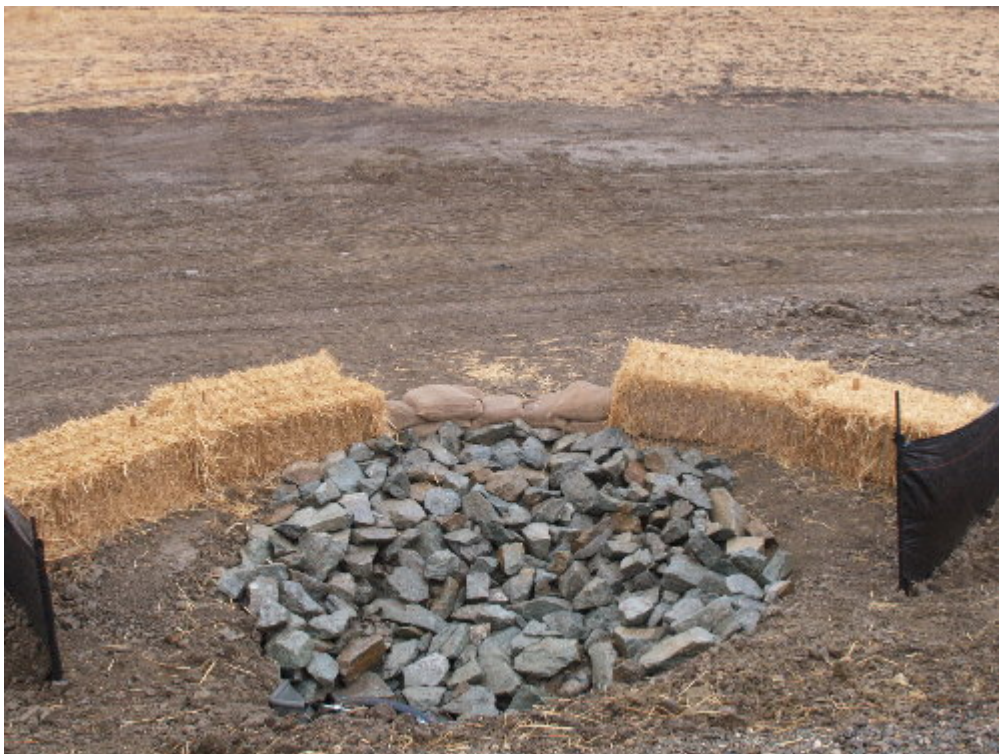
Figure 2 – Straw bales upstream of culvert installation along Moller Ranch Road.
