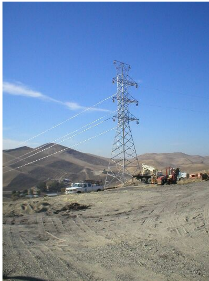
Figure 5 – Line pulling at tower 13 next to the Transition Station, November 17 th .
