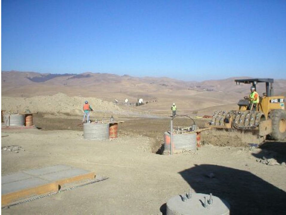
Figure 1 – Transition Station. November 18 th .
