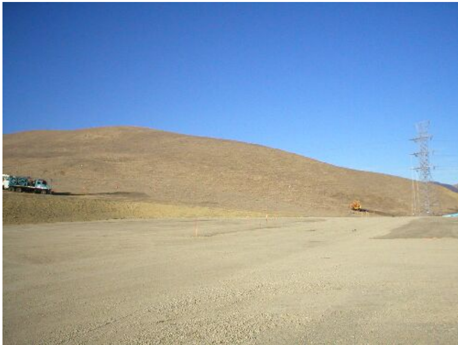
Figure 4 – Line pulling next to the Substation, November 17 th .
